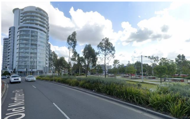
Figure 8 Castle Hill Metro Station and Arthur Whitling Reserve
