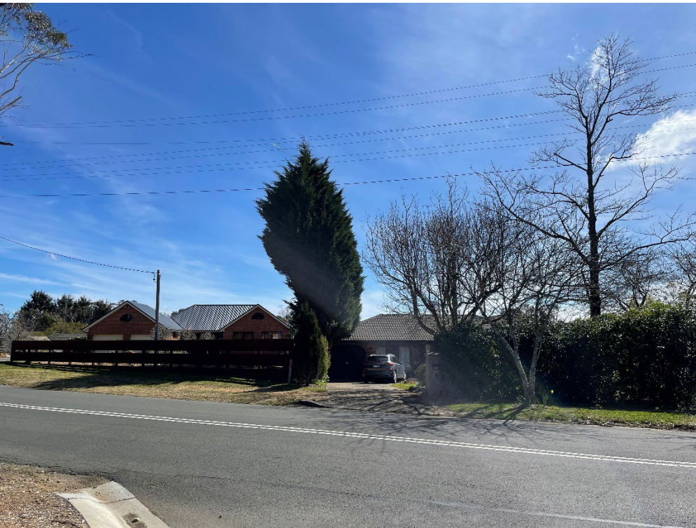
Photos 8 & 9 – Existing Services and Infrastructure
