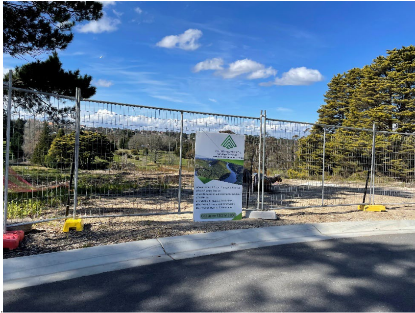
Photo 4 – Photo 4 – Site entry fencing and project signage (looking west)
