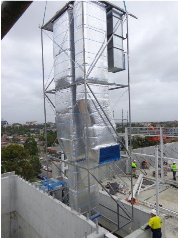
Figure 32: Examples of prefabricated services modules
