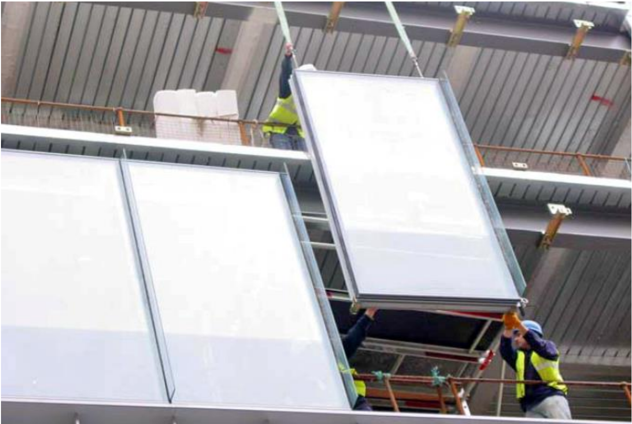
Figure 31: Typical curtain wall panel installation
