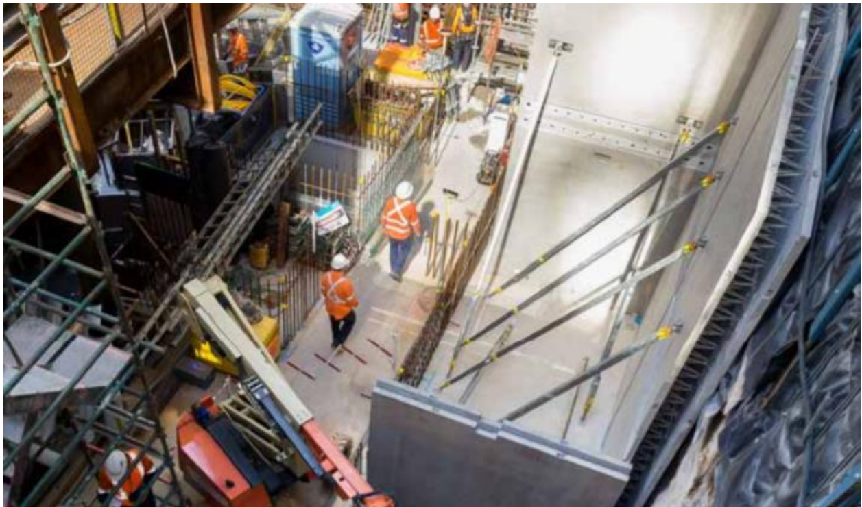
Figure 26: example of a double wall precast concrete panel
