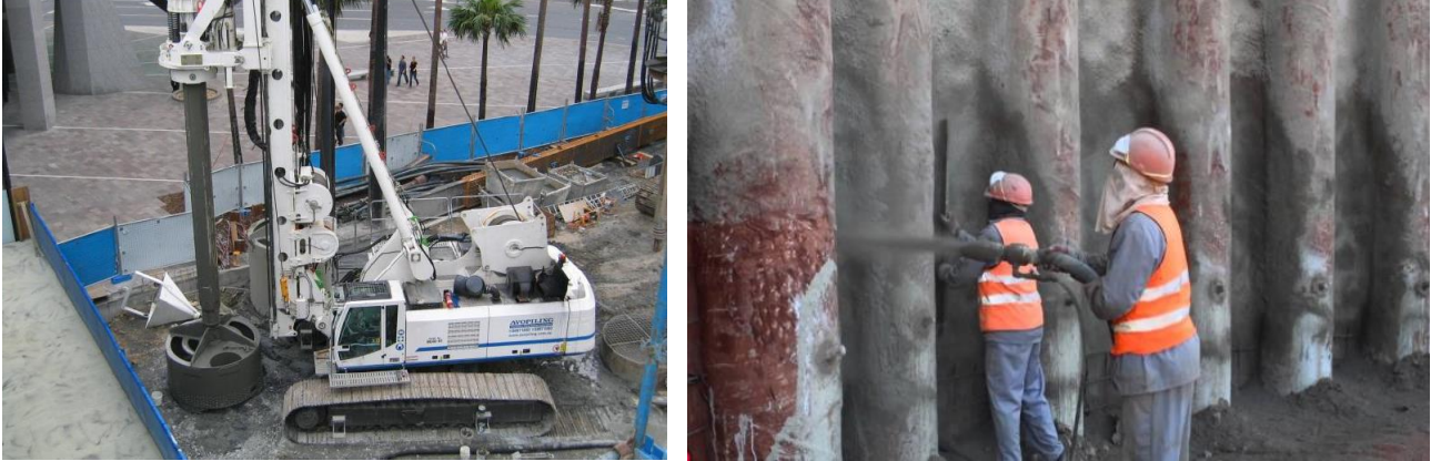
Figure 23: Examples of piling (left) and shotcreting (right) activities
