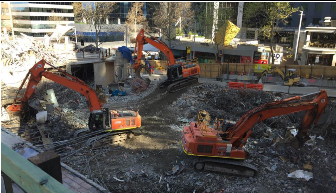
Figure 24: Example of excavation works
