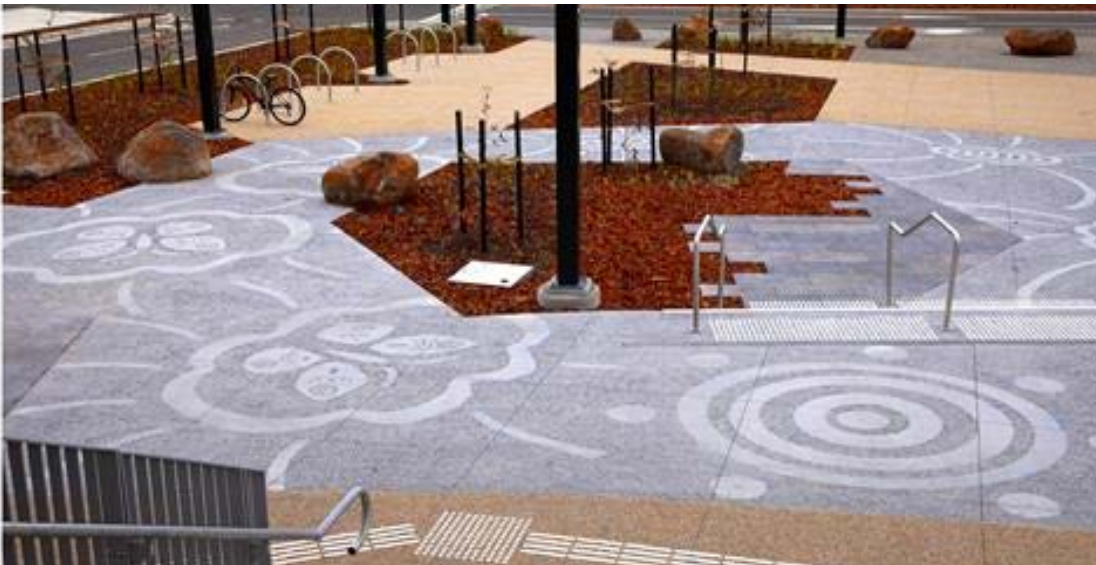
Ballarat Line Upgrade
