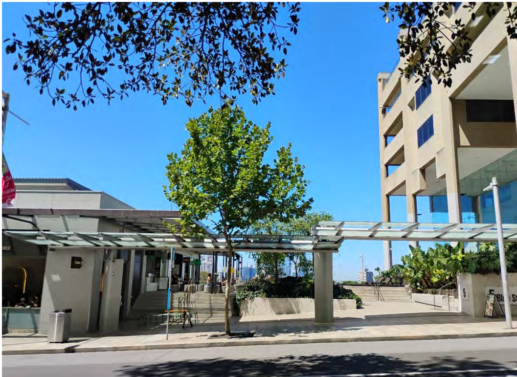
Photo 3: Photograph of the courtyard looking south
