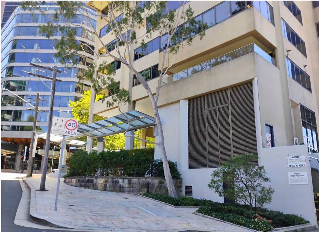
Photo 5: Photograph of the western portion of the Zurich building
