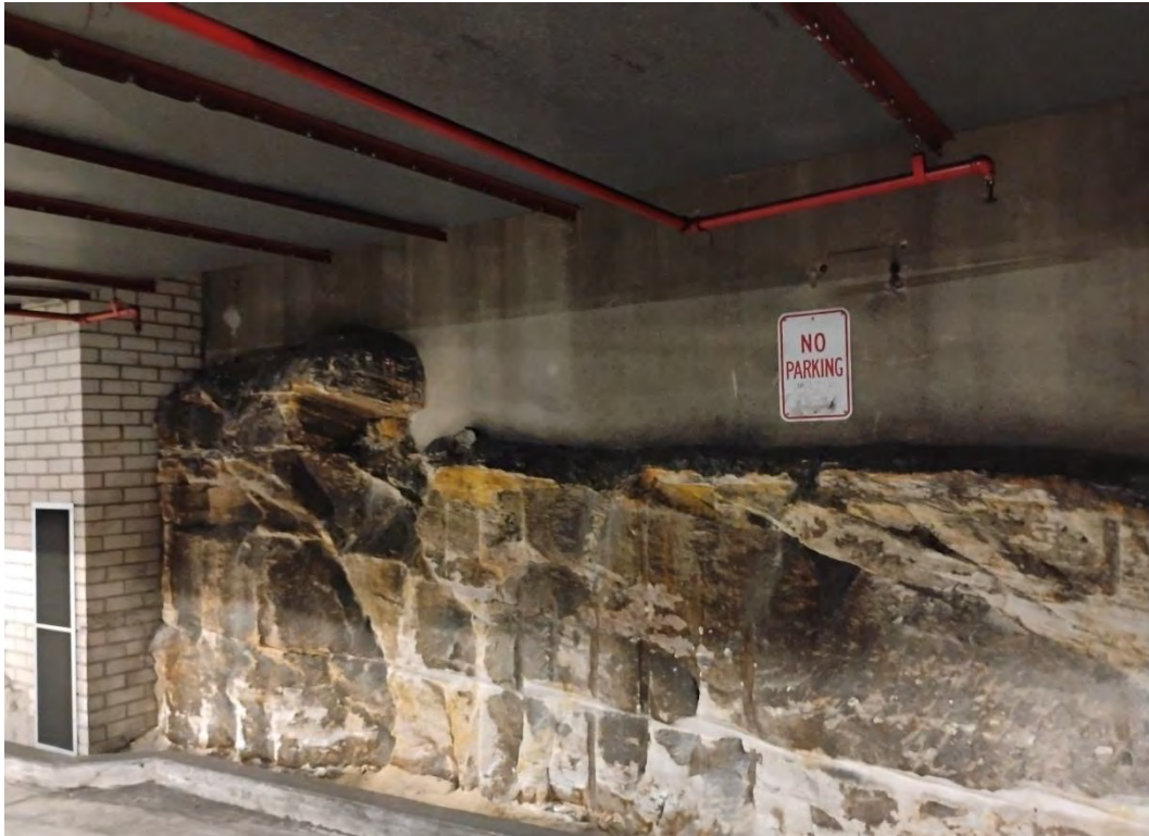
Photo 13: Photograph of the rock outcrop along the northern wall of the lower basement level
