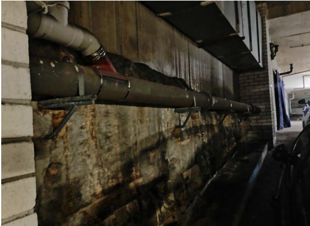
Photo 9: Photograph of the rock outcrop along the northern wall of the upper basement level
