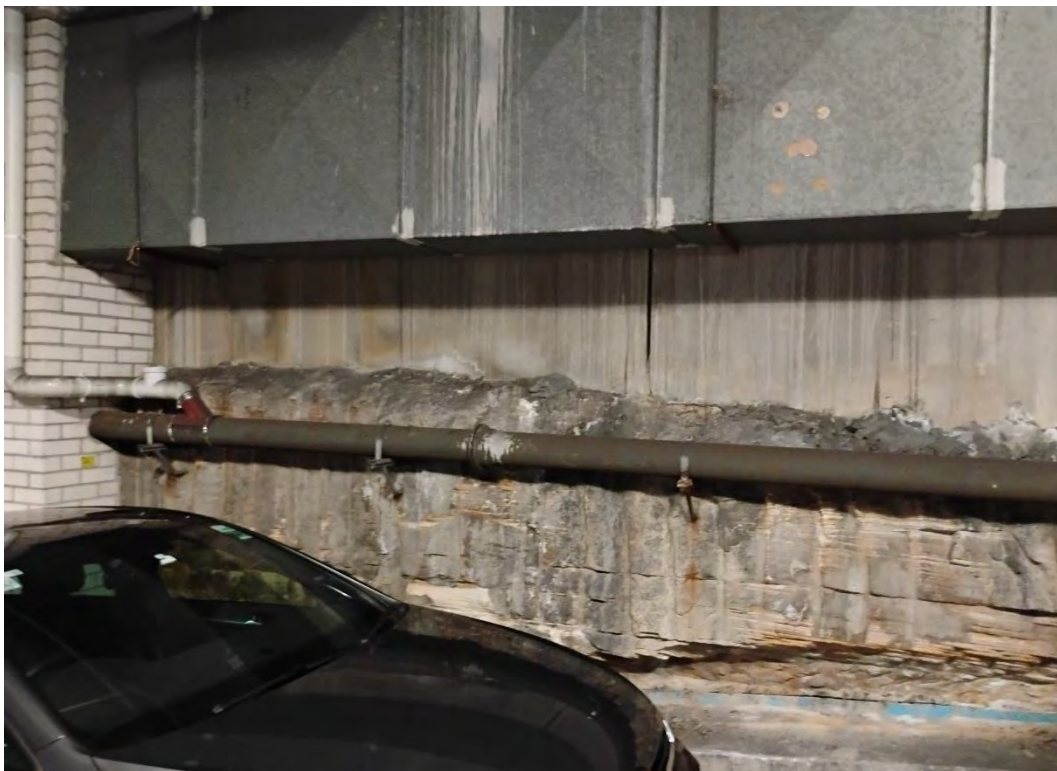
Photo 10: Photograph of the rock outcrop along the northern wall of the upper basement level
