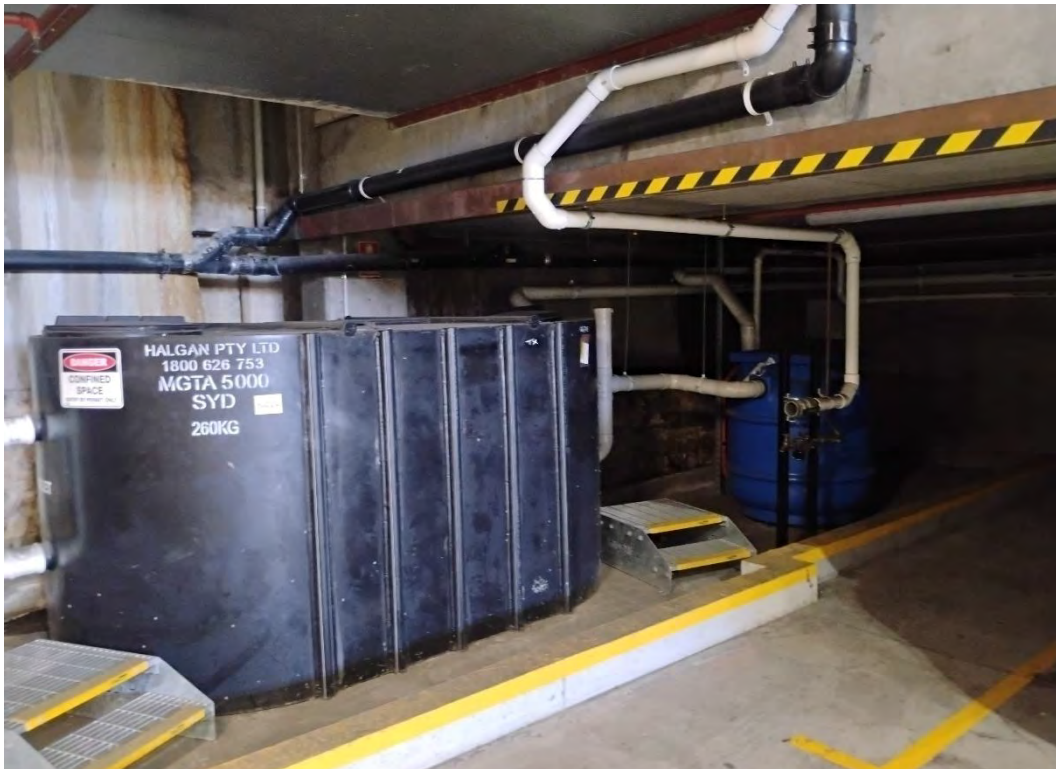
Photo 15: Photograph of the grease trap in the north-eastern corner of the lower basement level
