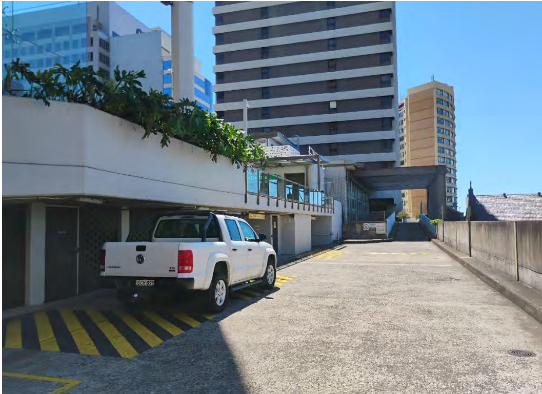
Photo 7: Photograph of the driveway with the courtyard above
