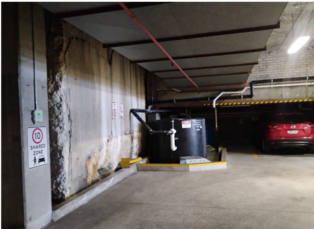
Photo 14: Photograph of the grease trap in the north-eastern corner of the lower basement level
