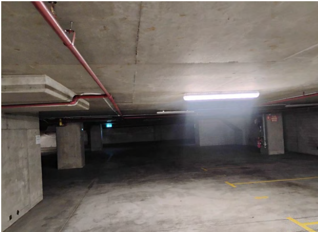
Photo 11: Photograph of the northern portion of the lower basement level
