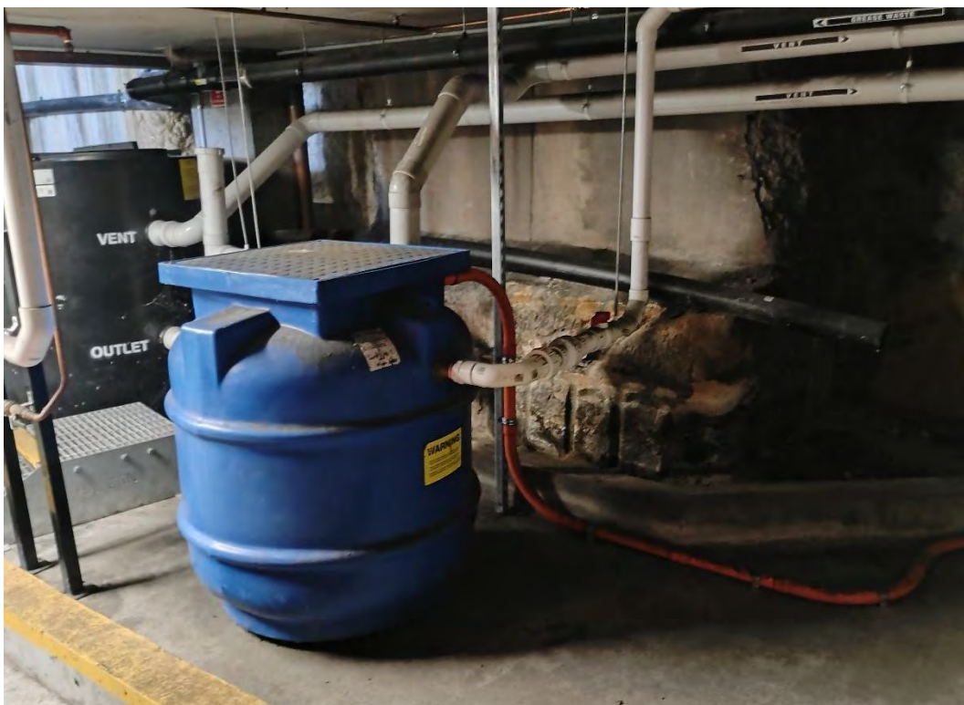
Photo 16: Photograph of the grease trap in the north-eastern corner of the lower basement level
