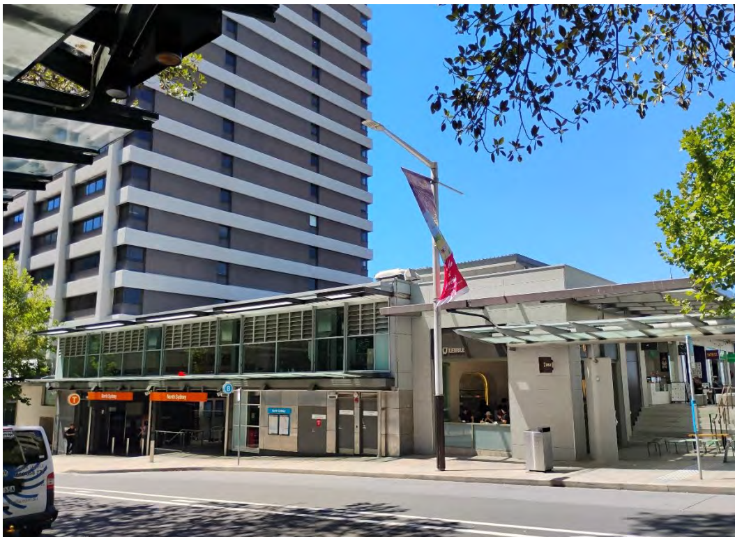
Photo 2: Photograph of North Sydney station looking south
