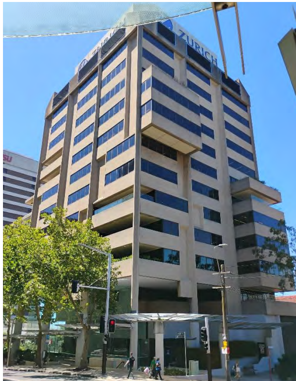
Photo 1: Photograph of the Zurich building looking south-east
