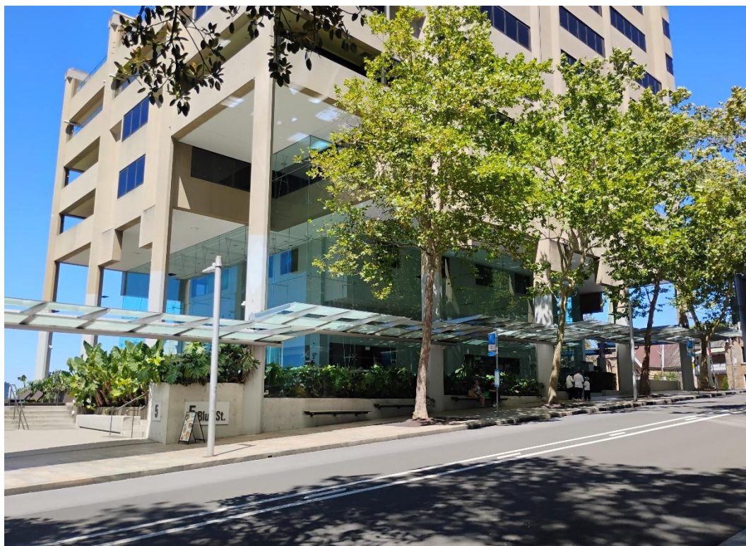
Photo 2: Photograph of the site at street level looking south-west
