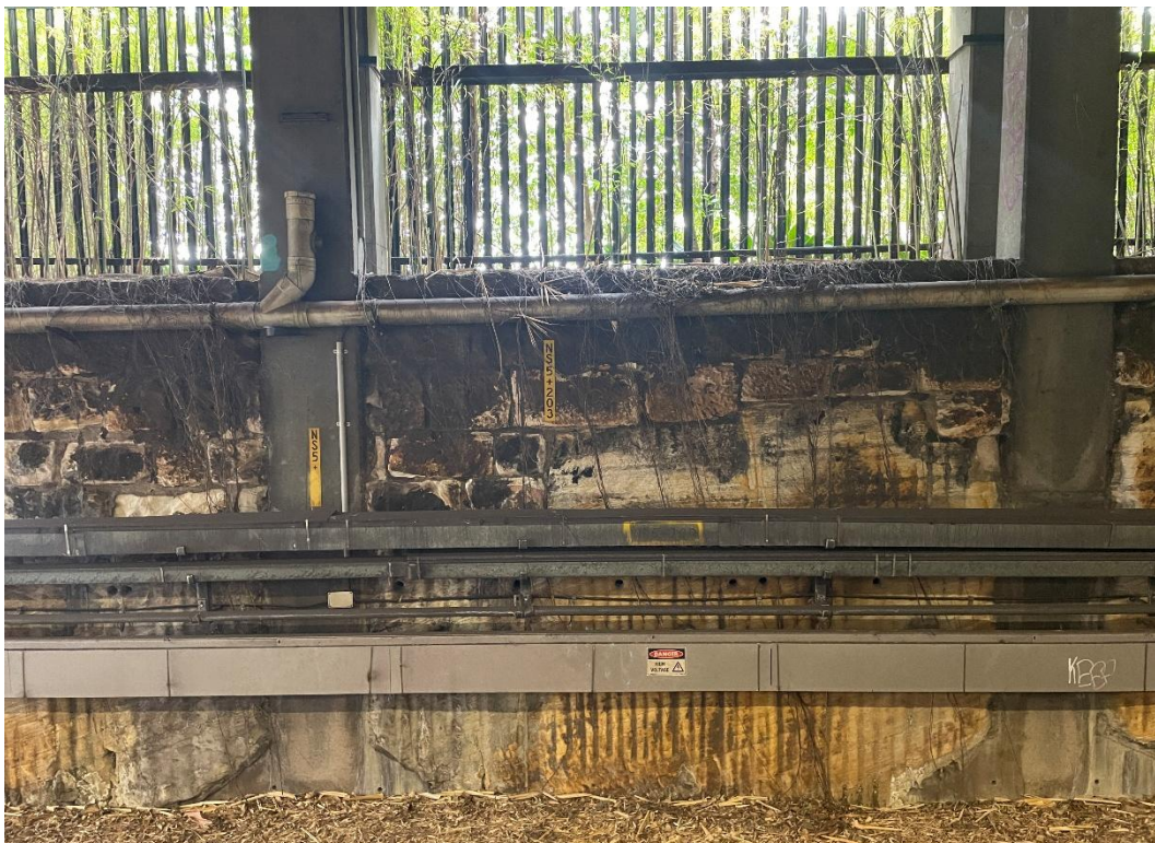
Photo 18: Photograph of the rock along the southern boundary from Platform 4 including the existing tapered foundations of the structure above
