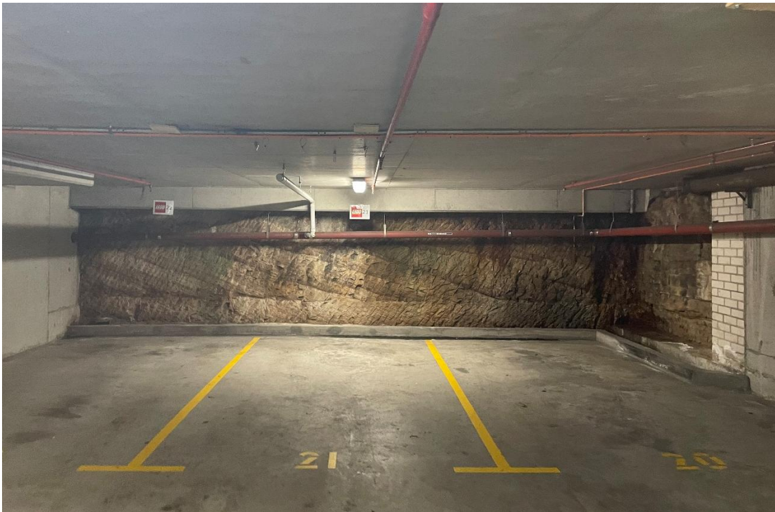
Photo 6: Photograph of the rock outcrop along the western wall (northern end) of the upper basement level
