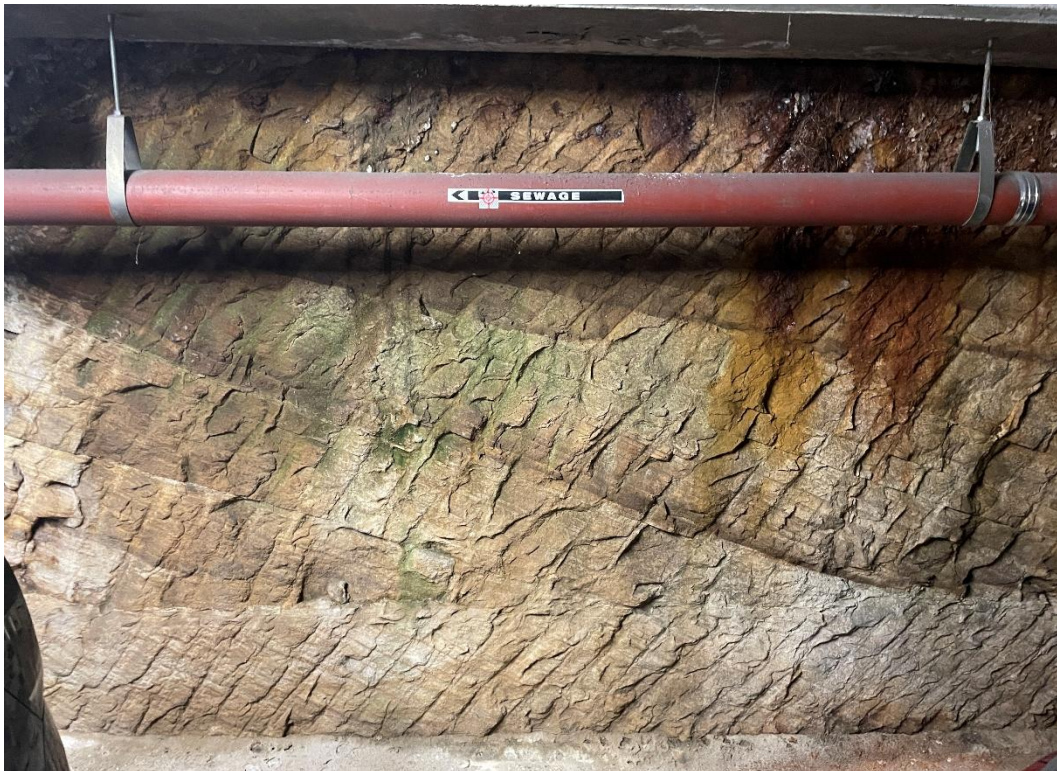
Photo 8: Photograph of the rock outcrop along the western wall of the upper basement level showing cross-bedding
