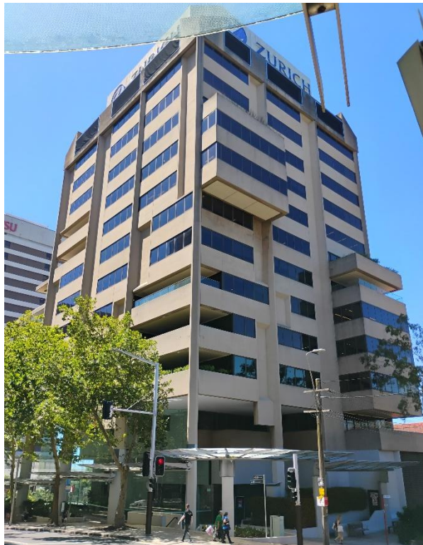
Photo 1: Photograph of the site looking south-east from the intersection of Blue Street and Blues Point Road
