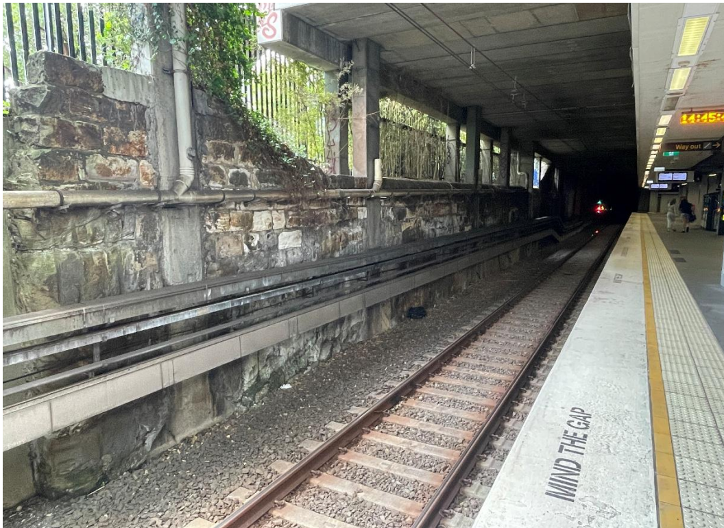
Photo 15: Photograph of the rock along the southern boundary from Platform 4 at approximately the eastern end of the site looking west
