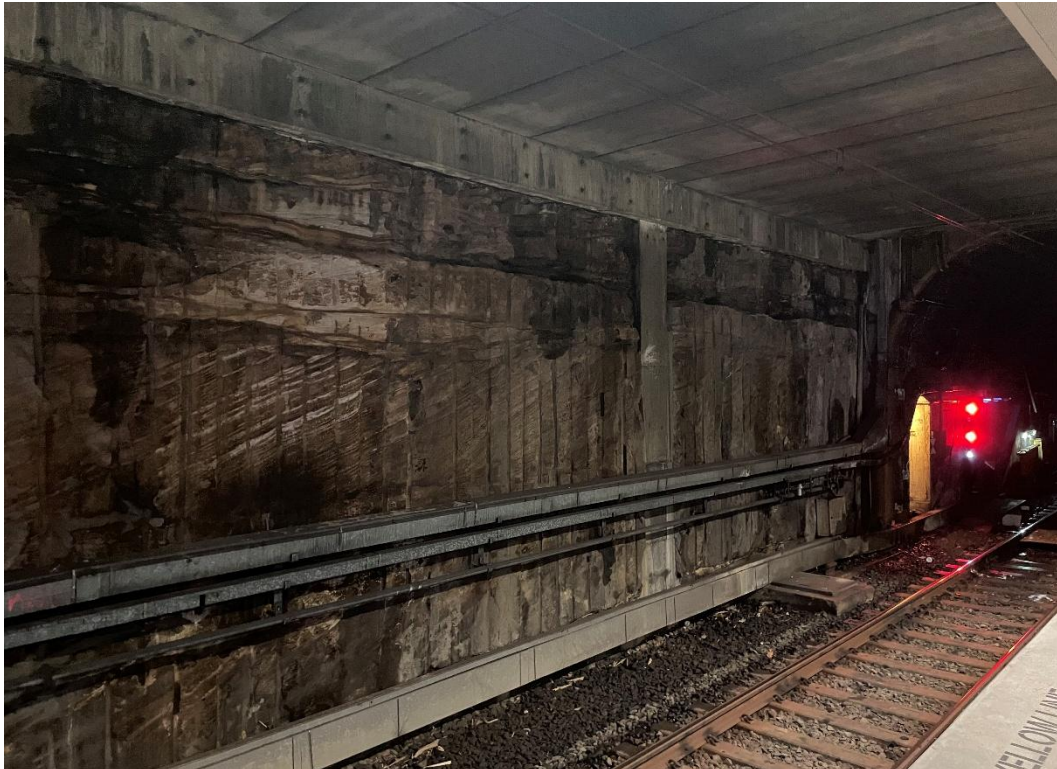
Photo 17: Photograph of the rock along the southern boundary and southern tunnel portal at the western end of Platform 4
