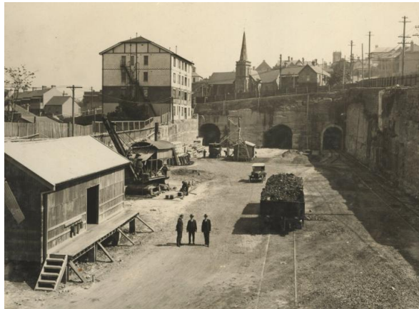
Figure 3.4: Construction of North Sydney Station 1925 – directly beneath the current study area, looking west Source: NSW State Archives NRS-12685-1-[4/8722]-4/8722-10
