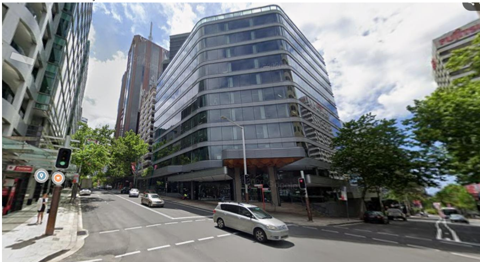
Figure 4-10: Looking north-east at the corner of Miller Street and Blue Street showing existing high density commercial development characterising the southern portion of the North Sydney CBD. Source: Google Streetview accessed May 2026.
