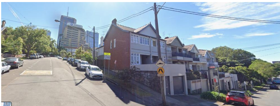
Figure 4-16: Looking north from the corner of Miller Street and Lavender Street towards the subject site illustrating the lower density historic fine grain character of the Lavender Bay HCA located to the south. Source: Google Streetview accessed May 2026.
