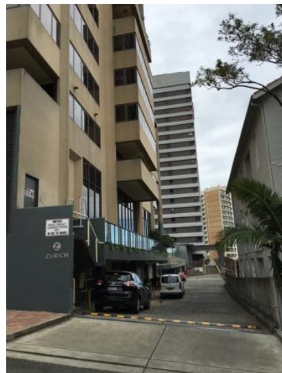
Figure 4-6: View of existing service lane and southern elevation. Source: FJC Architects.
