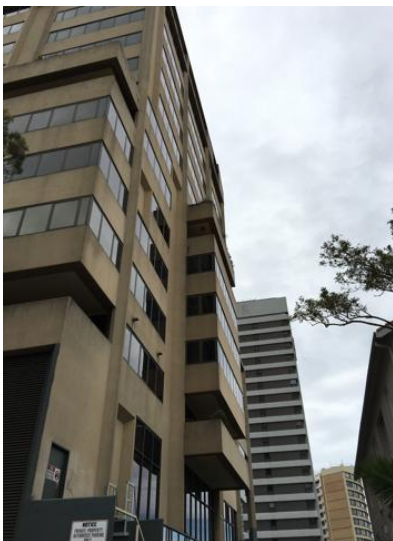
Figure 4-5: View of existing southern elevation Source: FJC Architects.
