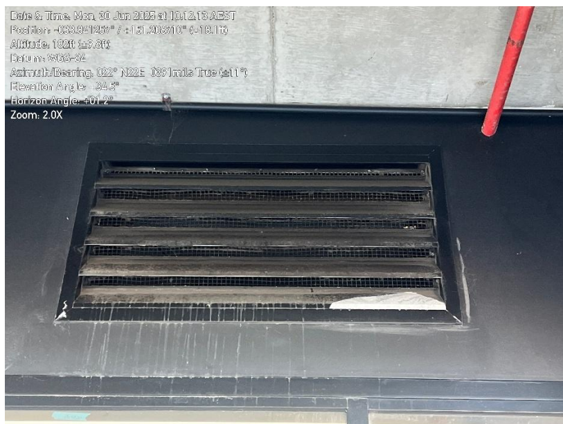
Photo F5: View outside in the carpark showing a mesh screen which would be preventing bats from entering the building
