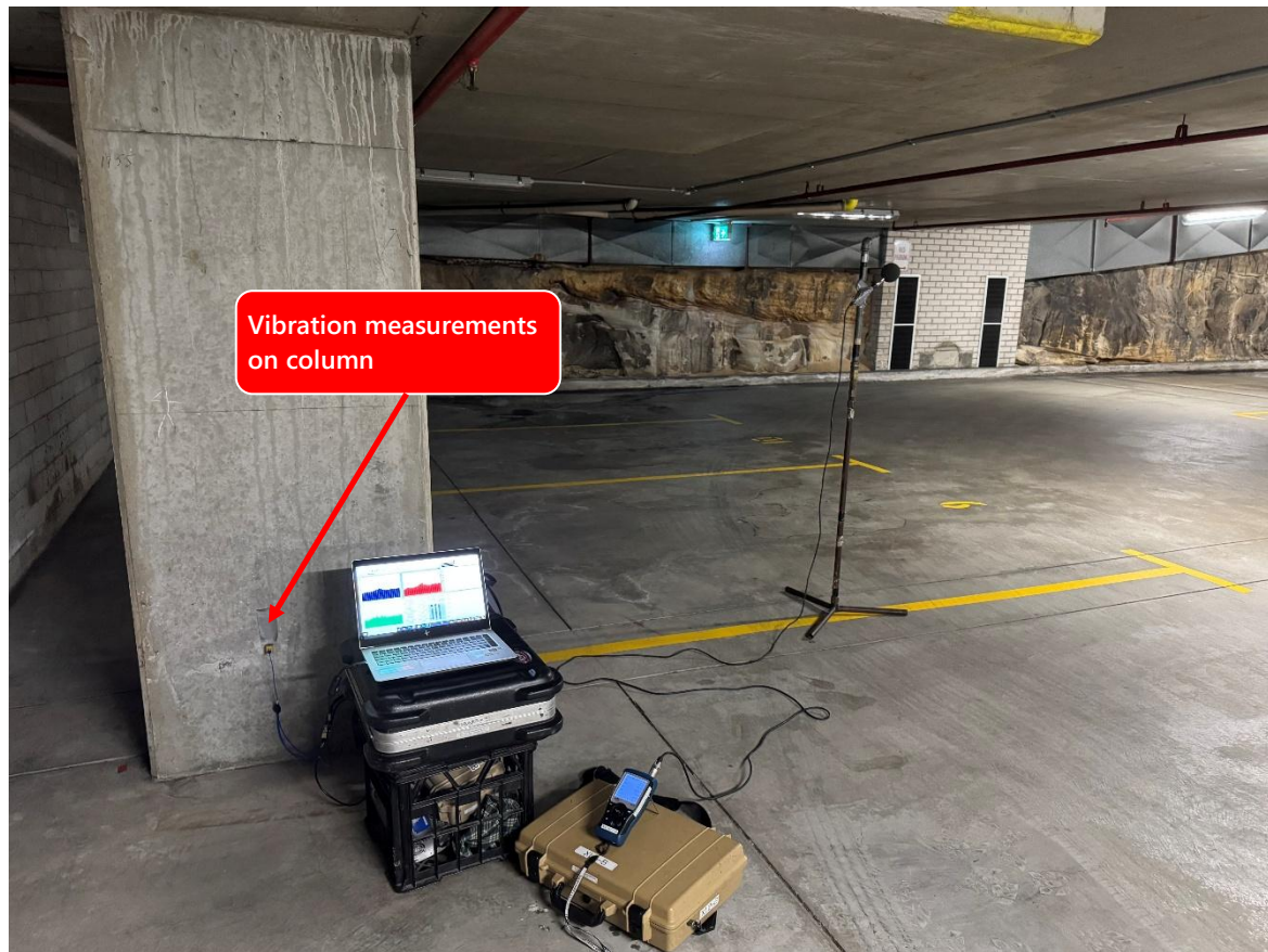
Figure 6-1: Vibration measurement location in carpark – above Platforms 1 and 2
