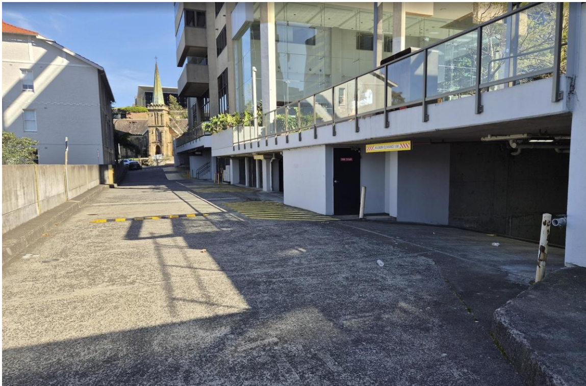
Figure 4 Existing Phillips Lane
