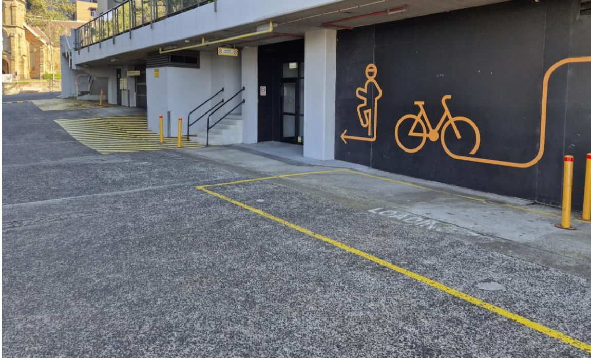
Figure 14 Existing loading bay on Phillips Lane
