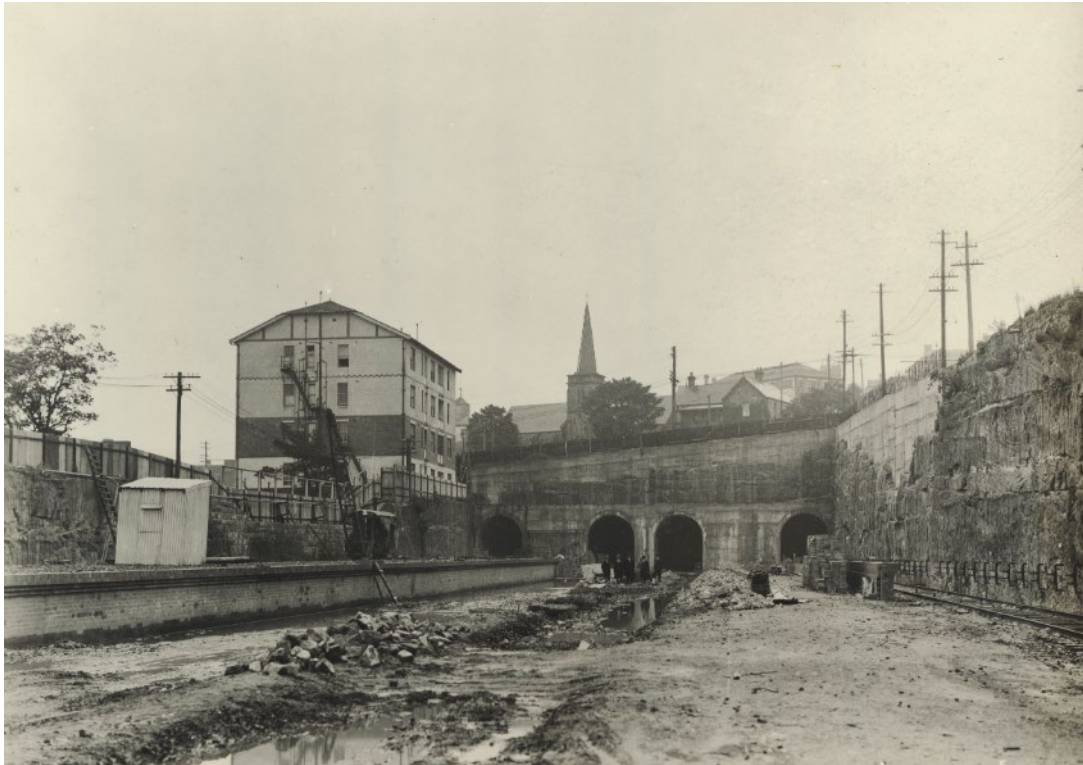
Figure 3.5: Construction of North Sydney Station 1931 – directly beneath the current study area, looking west Source: NSW State Archives NRS-12685-1-[4/8723]-4/8723-9
