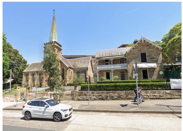
West of the Site – St Peter's Presbyterian Church as viewed from Miller Street
