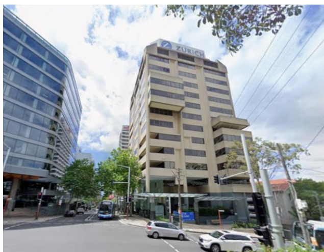
View of the Site from Blue Street, to the Site's West
