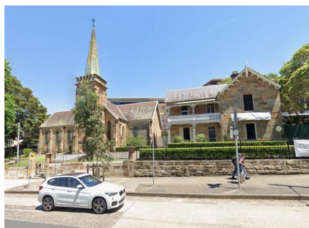
West of the Site – St Peter's Presbyterian Church as viewed from Miller Street
