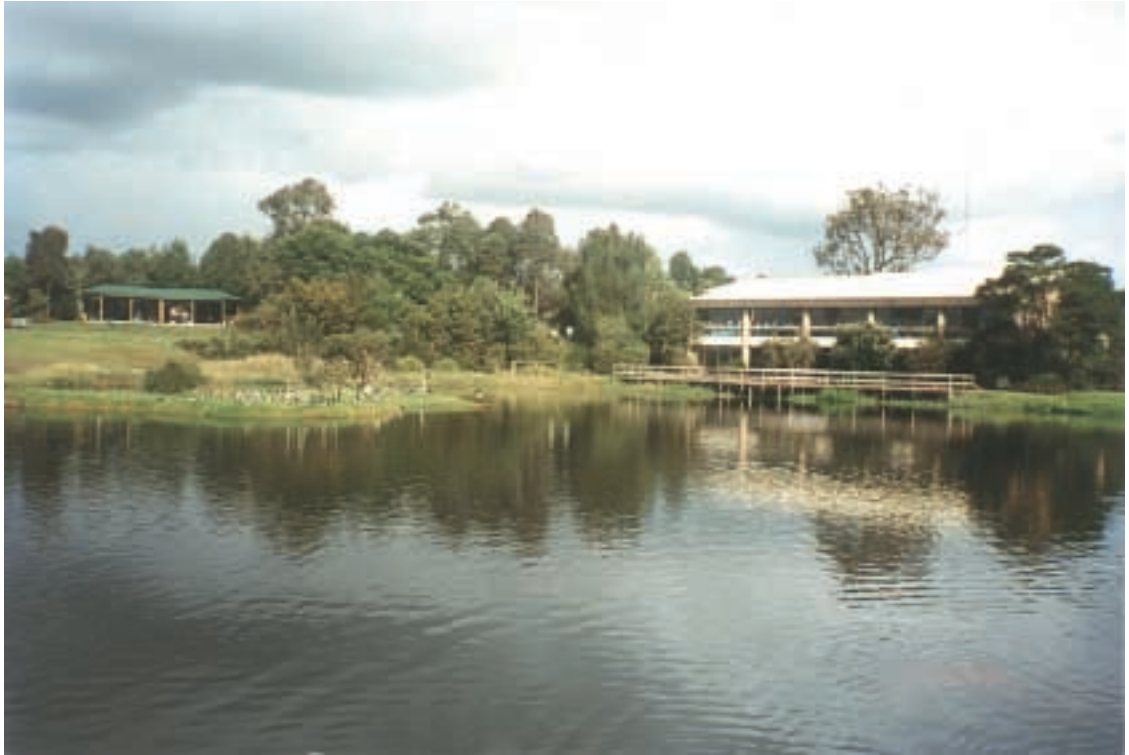
Environmental Education Centre at Shortland Wetland Centre
