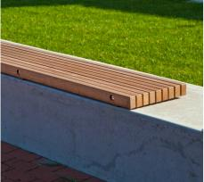
IN SITU CONCRETE SEATING WALL with timber battens Concrete: Plain Grey Timber: 125x38mm Hardwood 'Blackbutt'
