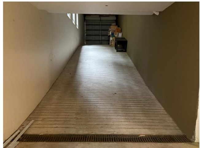
Plate 35. View north-east. Underground garage beneath house showing sloped driveway and subfloor storage/parking area
