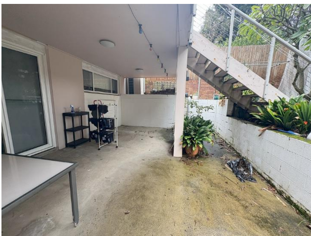
Plate 48. View south-east showing basement level concreted area and retaining walls.
