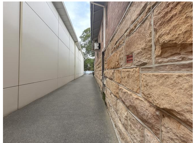
Plate 29. View north-east along the sloped driveway highlighting gradient from street frontage to rear yard.
