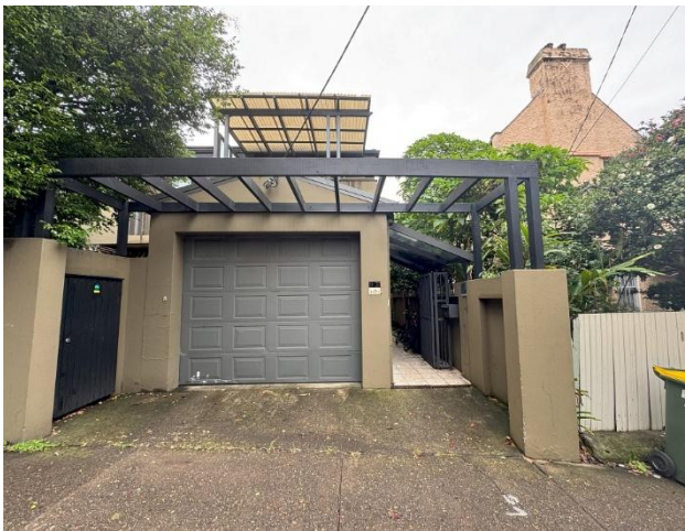
Plate 34. View south-west. Front view of 27A-B Dover Road, showing garage entry and rendered boundary walls.
