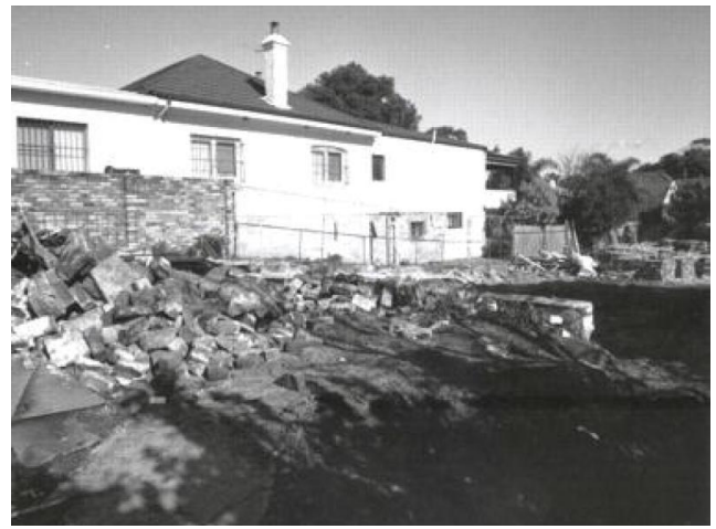
Plate 21 Site after the demolition of Overdale, 1994. 36
