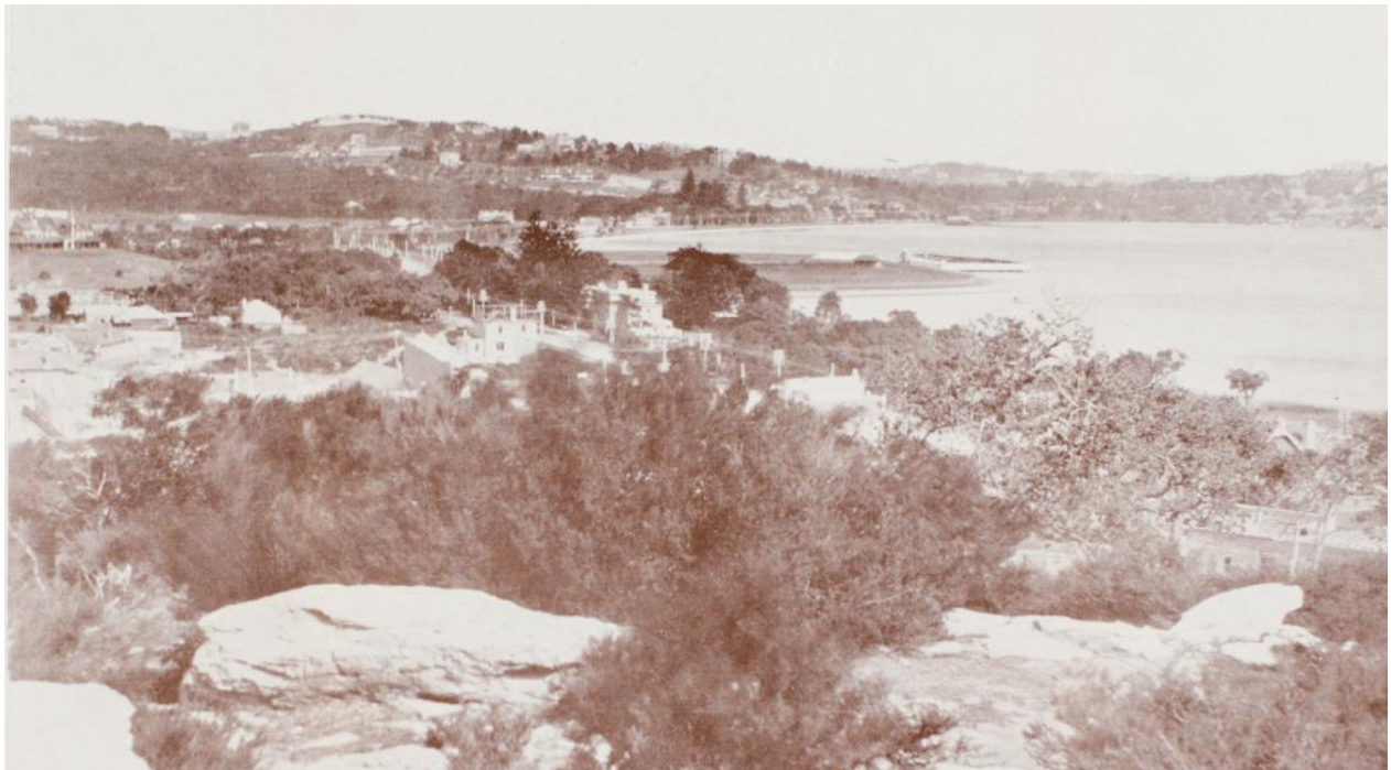
Plate 9 The Mitchell Estate, north of the site, showing view of Rose Bay prior residential subdivision and development, c1910.
