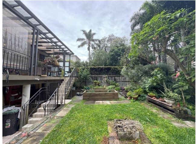
Plate 37. View south-east across backyard showing elevated rear garden, terraced retaining walls, and foundational pylons.
