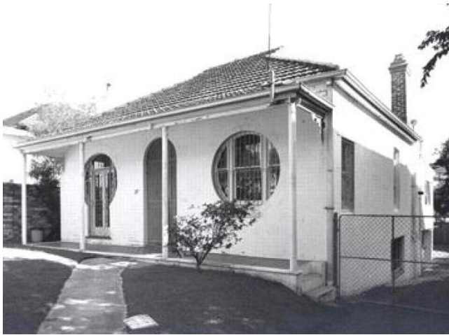
Plate 20 Overdale in 1994 just before its demolition. 35
