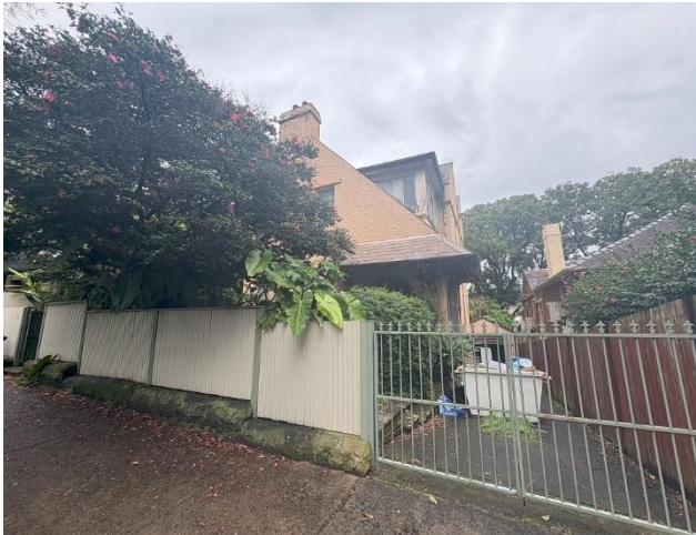
Plate 30. View south-west showing the front facade.
