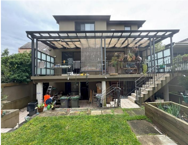
Plate 36. View north-east. Rear façade of dwelling and backyard, showing concrete retaining wall, raised garden, and foundational pylons.
