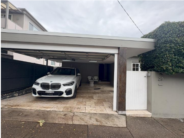
Plate 40. View south-west. Front facade of 29Dover Road, showing driveway and pedestrian entryway.
