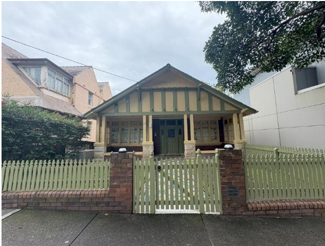
Plate 26. View south-west. Front facade of 23 Dover Road, showing Federation-era dwelling and front setback.
