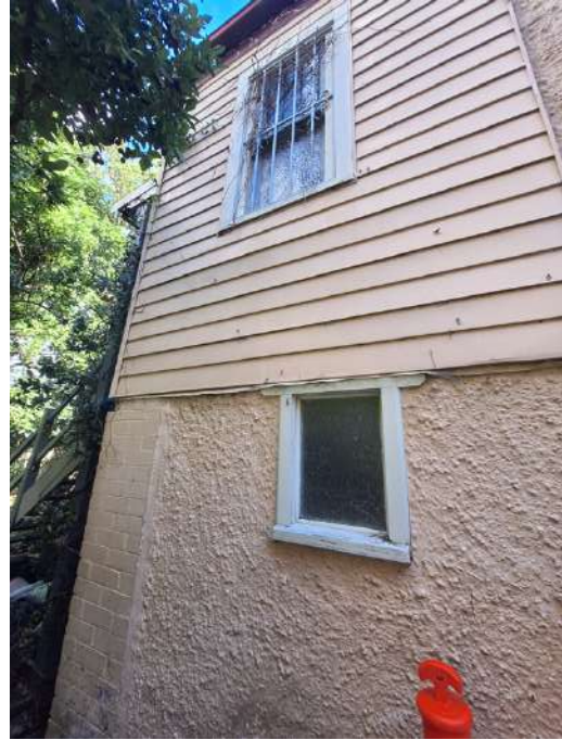
Figure 27: Detailed view of the weatherboard extension on tall brick piers at the rear of No. 25 Dover Road, Rose Bay
