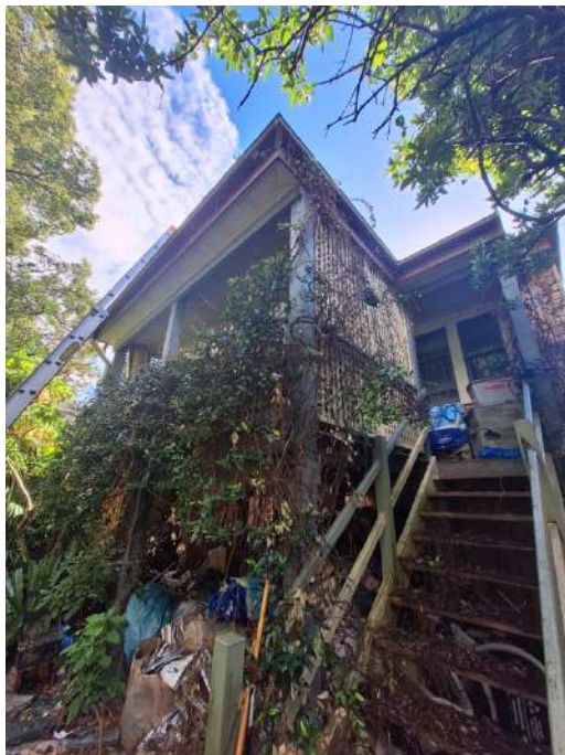
Figure 28: The verandah of the rear extension of No. 25 Dover Road, Rose Bay.
