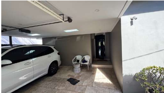
Figure 59: The front elevation of No. 29 Dover Road, Rose Bay underneath the carport.
