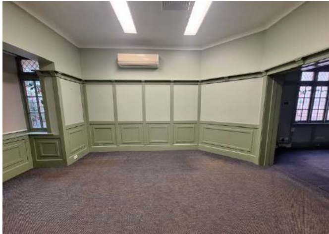
Figure 14: The waiting room of No. 23 Dover Road, Rose Bay showing the modern carpet flooring, timber wall panelling and modern plasterboard ceiling.
