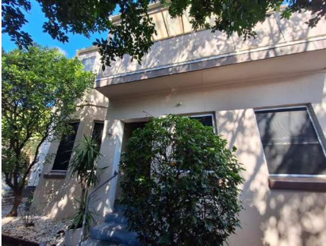
Figure 72: The front elevation of No. 31 Dover Road, Rose Bay.
