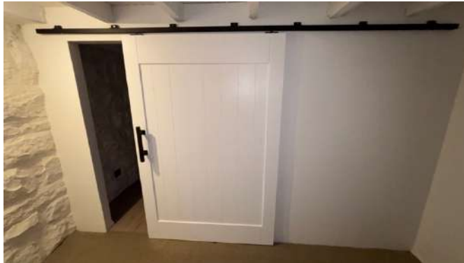
Figure 68: The large barn door and painted sandstone of the basement area.
