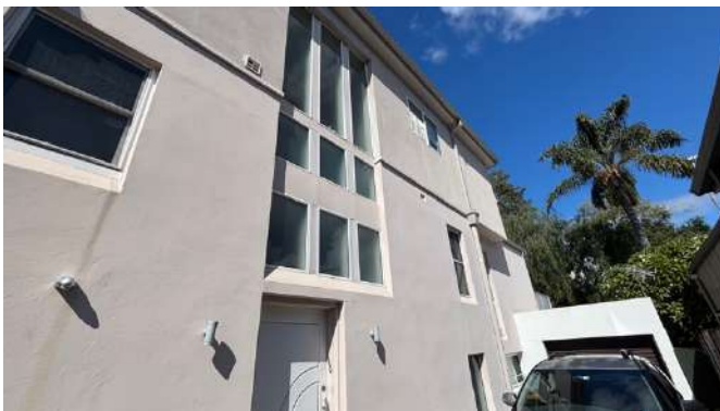
Figure 74: The large glazing feature above the front entrance to the rear unit of No. 31 Dover Road, Rose Bay.
