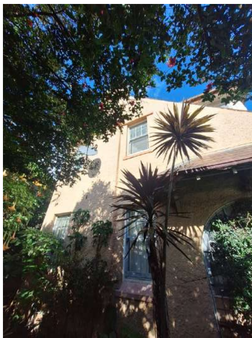
Figure 24: The front elevation of No. 25 Dover Road, Rose Bay.
