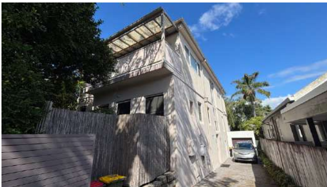
Figure 73: The northern elevation of No. 31 Dover Road, Rose Bay.
