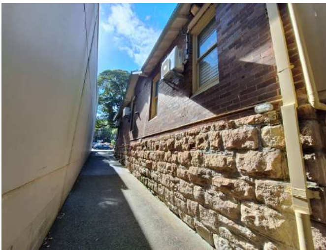
Figure 11: The northern elevation of No. 23 Dover Road, Rose Bay.
