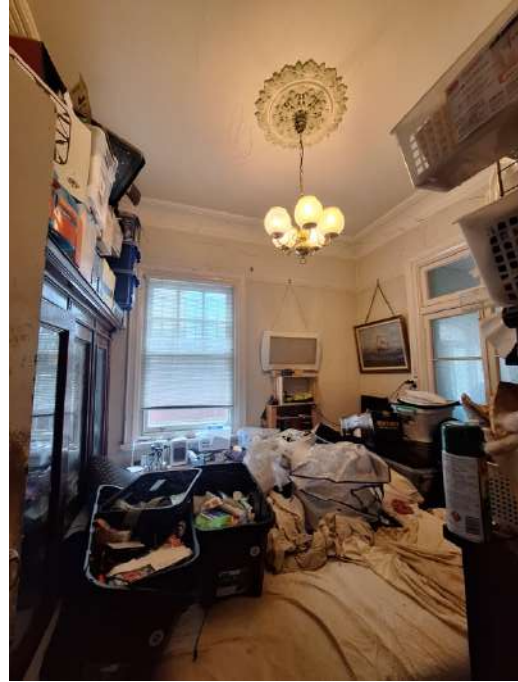
Figure 32: A smaller room on the ground floor showing a simpler ceiling with a plaster ceiling rose, as well as the timber architrave and toplight of some of the internal doors.
