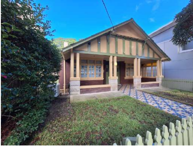
Figure 10: The front of elevation of No. 23 Dover Road, Rose Bay.
