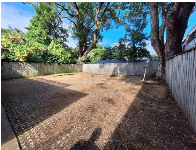
Figure 9: The carpark in the rear yard.
