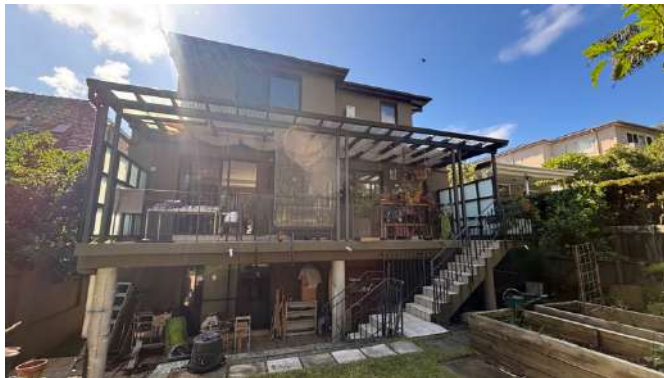
Figure 45: The rear elevation of No. 27 Dover Road, Rose Bay.
