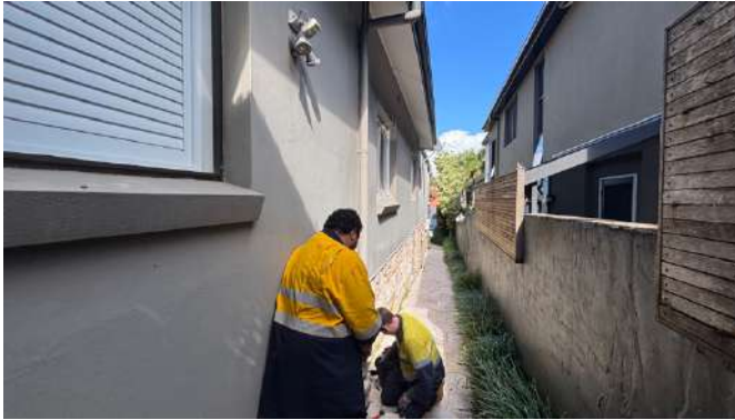
Figure 56: The path in the northern setback linking the front and rear yard.
