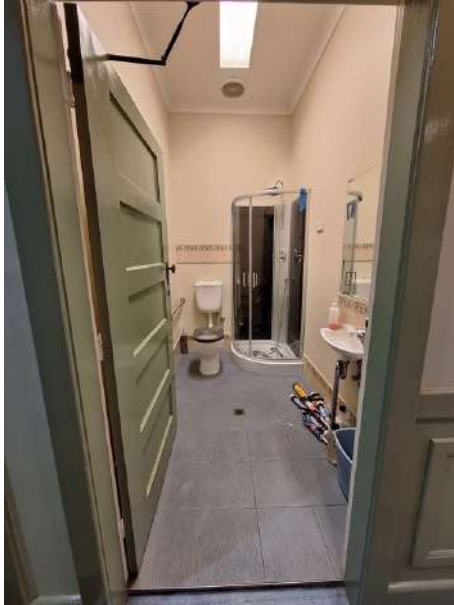
Figure 18: An example of one of the bathrooms which shows the modern fit out of the bathrooms in the building.
