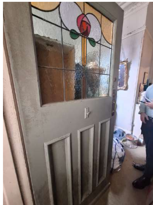
Figure 29: The timber and glass front door.
