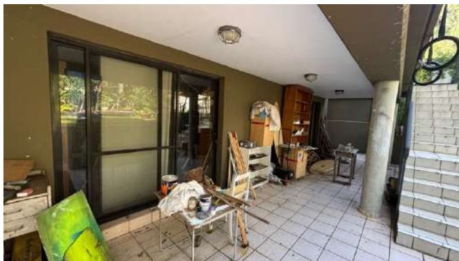
Figure 46: The rear elevation of the lower ground floor.
