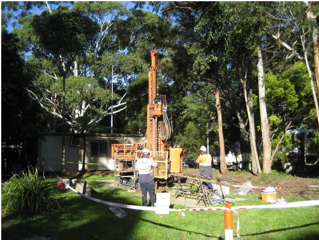
Photo 14: Drilling of borehole CBH03 in the north-western part of the site.
