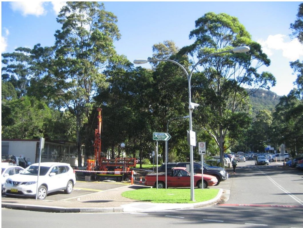
Photo 1: View (east to west) of existing carpark located at north-east corner of the site. Drilling rig set up over Borehole CBH01. Access road to western carpark on right side of photo.
