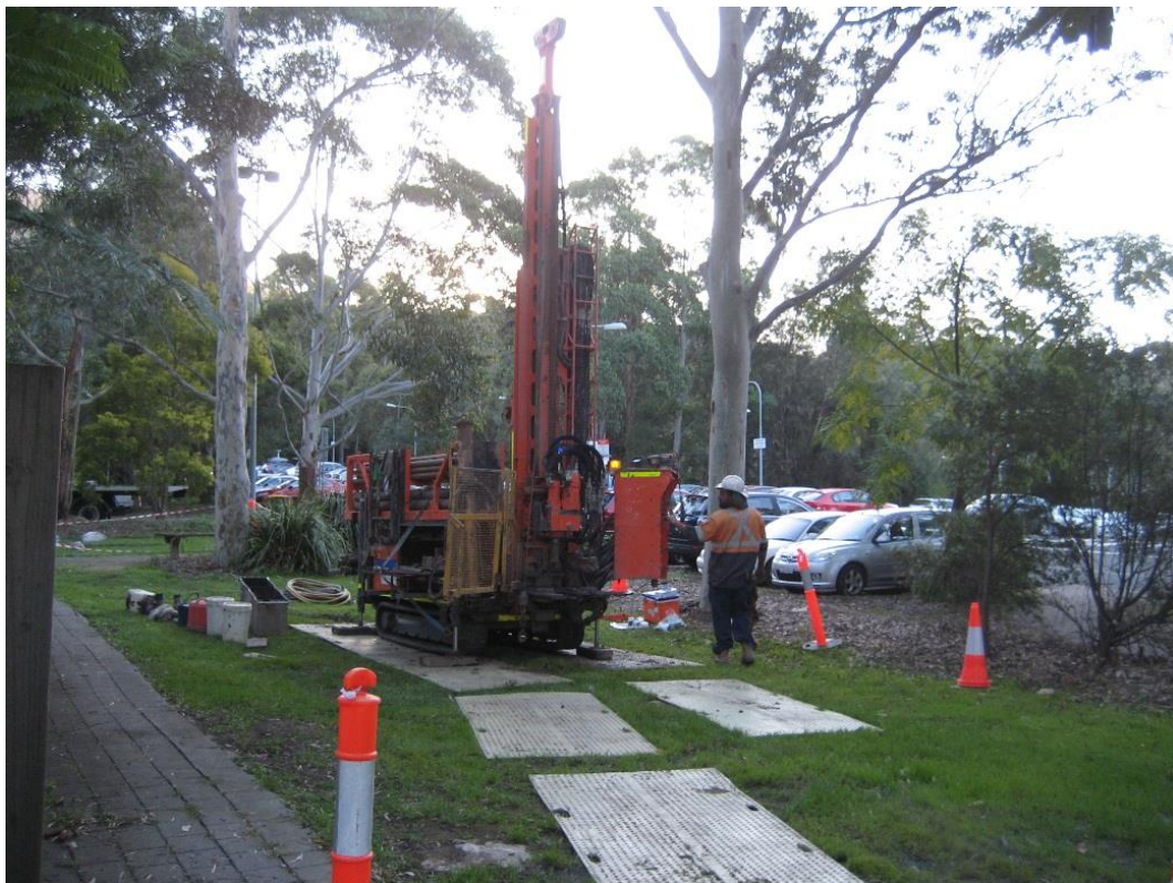
Photo 13: View of the borehole CBH02. Rigid mattresses used to minimise the damage to the grass.
