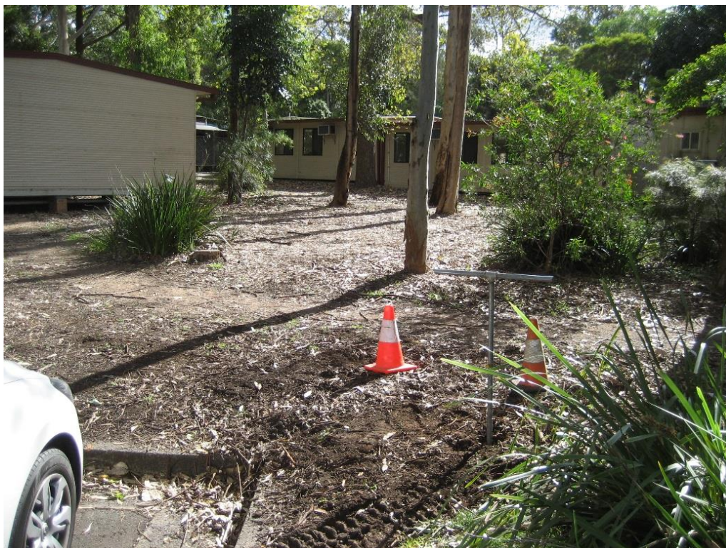
Photo 17: View of the borehole CBH06 near existing carpark (concrete slab- possible pit). Due to unusual resistance near the ground surface, borehole was drilled only by hand auger and terminated at 0.25m.
