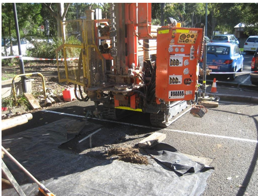
Photo 11: View of the borehole CBH01, drilled using hand auger prior to auger drilling.
