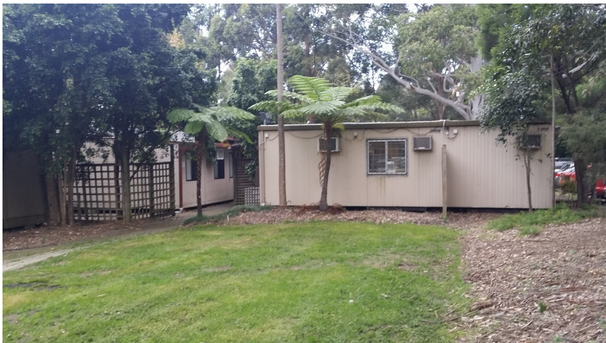
Photo 1 – Example of classroom (Classroom 50) as viewed from the north
