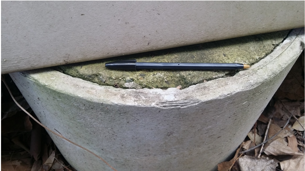
Photo 5 – Example of fibro encased concrete pier (at Classroom 54)
