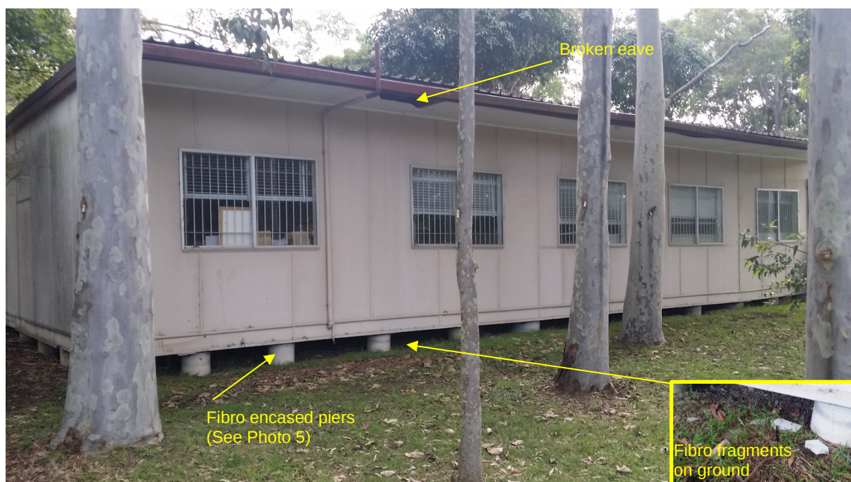
Photo 2 – Classroom 54 facing north west
