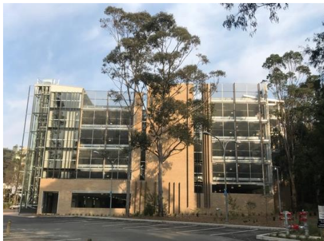
South Western Car Park P3 located south of the site
