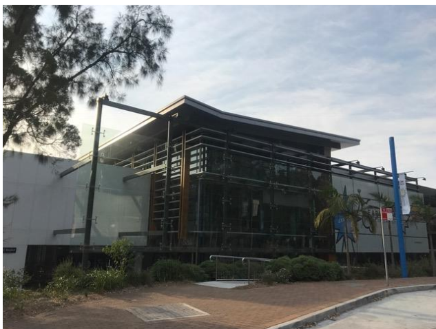
Early Start Facility looking south west from the site
