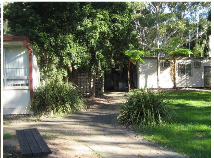
Existing demountable buildings viewed from the north
