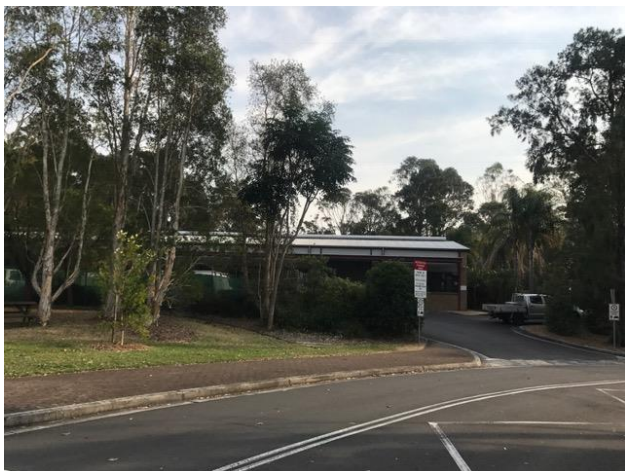
Facilities management building located north of the site
