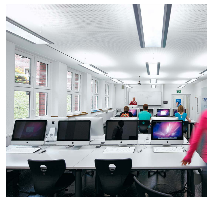
3 Suspended direct / indirect pendants to offices
