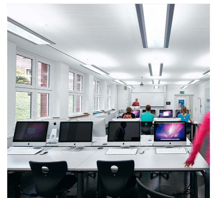
3 Suspended direct / indirect pendants
