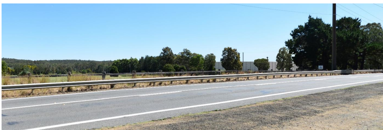
Figure 5-14 Detail of Figure 5-13 showing the noise barriers visible in breaks in the vegetation barrier due to tree removal
