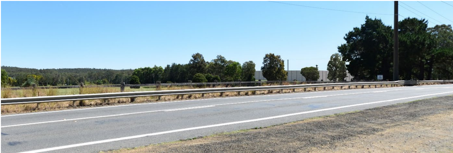
Figure 6.6-15: VP04 – Wine Country Drive southern view - detail of Figure 6.6-14 showing the centre of the proposed view, with the battery units and noise barriers visible extending from behind vegetation in the middle ground of the view
