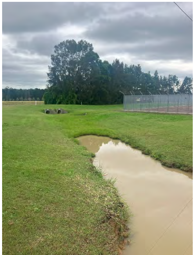
16 Looking northwest down the drainage easement towards Black Creek.
