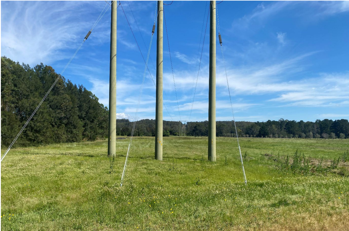
Figure 3: Looking west from site entry road, existing vegetation screen along Old North Road (left)
