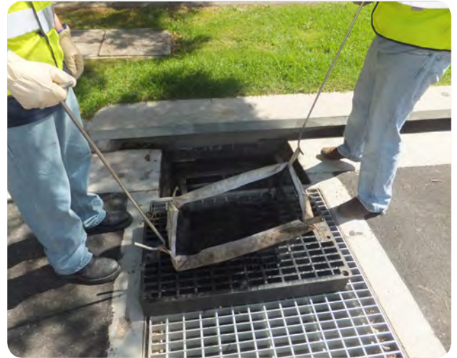
Photo 19 Reinstall filter bag
