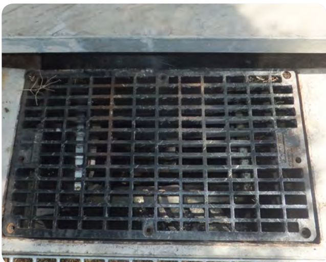
Photo 22 Installed filter bag and sealed pit
