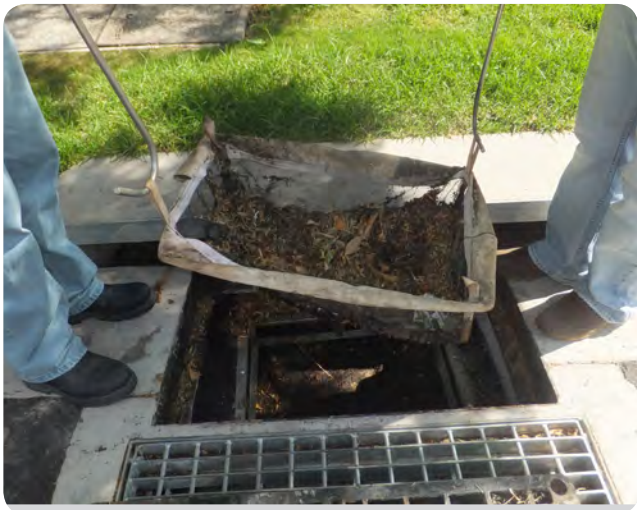
Photo 14 Lift the bag from the stormwater pit
