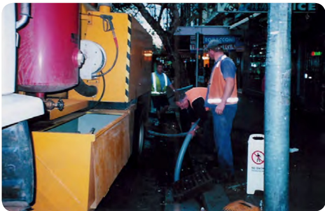
Photo 11 Cleaning an EnviroPod using the inductor method
