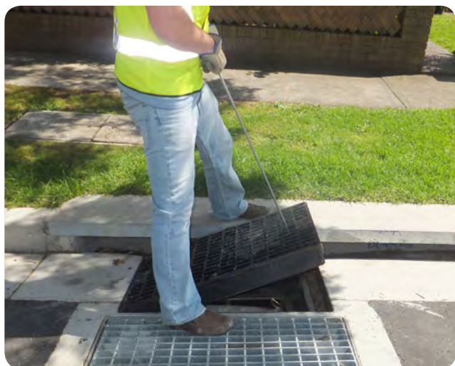
Photo 3 Lifting the grate
