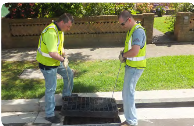
Photo 9 Lift grate above the support frame
