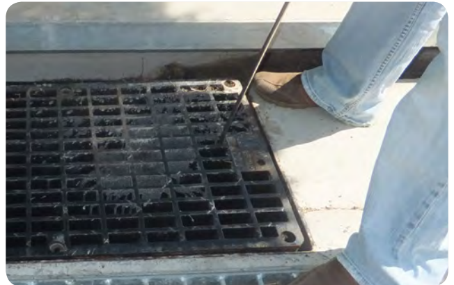
Photo 6 Insert hook near edge of grate
