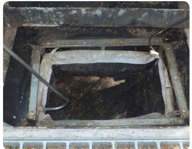
Photo 21 Correctly installed filter bag
