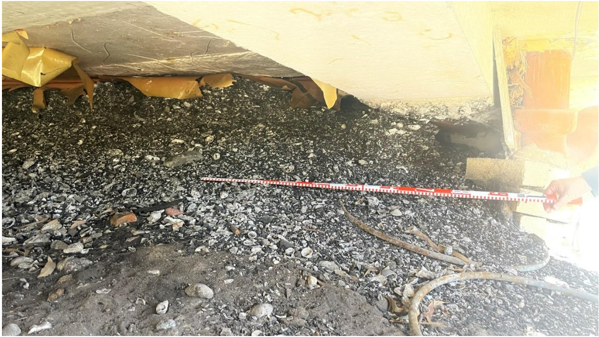
Plate 3. Plastic layer between dredged shell and building. (Source: Heritage Now 2024)
