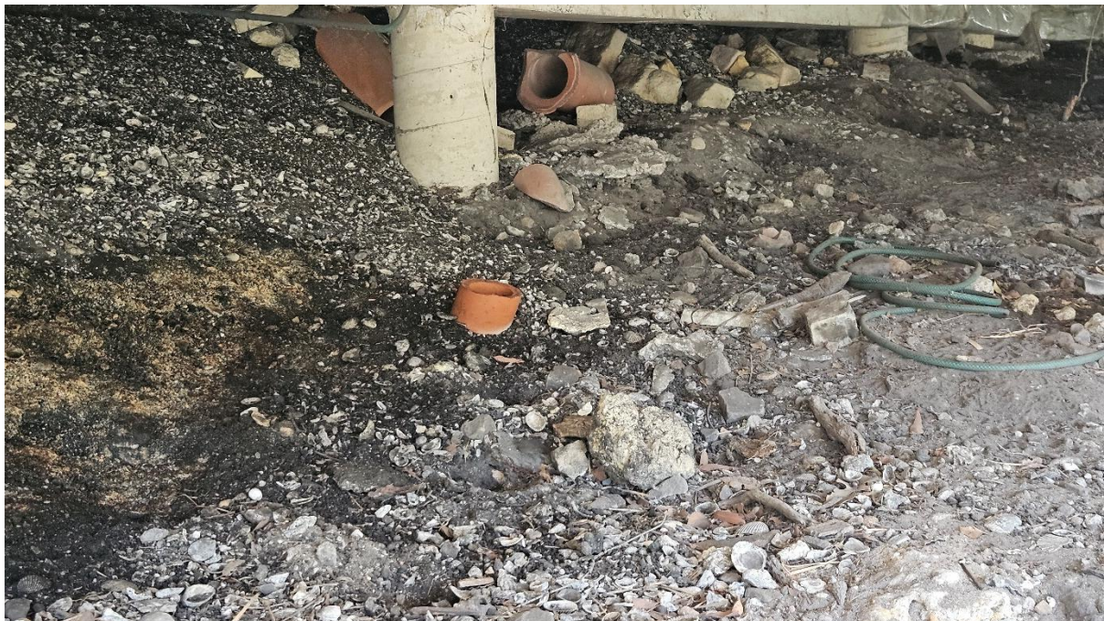
Plate 6. Dredged shell and imported grey sand intermixed with building rubble and sandstone pieces. (Source: Heritage Now 2024)
