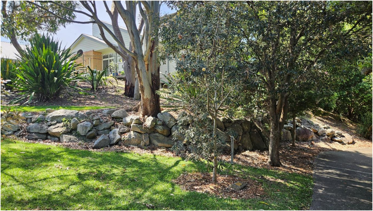
Plate 19. Sandstone used as a garden retaining wall. (Source: Heritage Now 2025)
