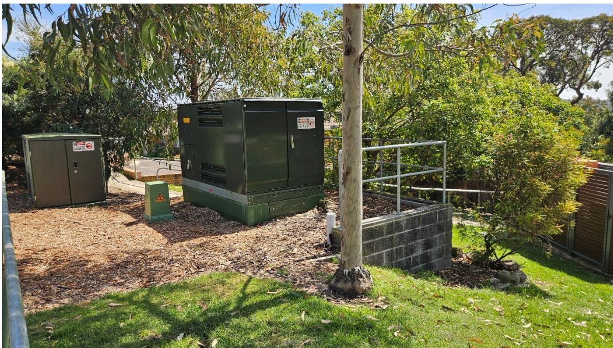
Plate 22. A retaining wall used to support a modified and infilled area. (Source: Heritage Now 2025)
