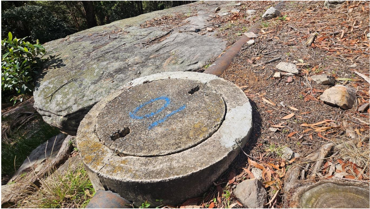
Plate 27. Overground water pipeline constructed into the roof of the rock shelter. (Source: Heritage Now 2024)
