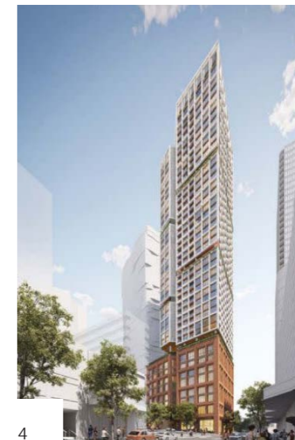
4 Telstra Exchange (BTR Residential) DKO Architects
