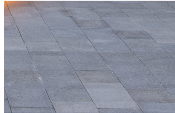
Paving on pedestals
