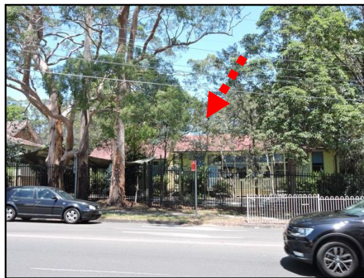
Figure 6. View to the northern boundary of the site, across Edgeworth David Avenue, facing south. Building J is indicated by the red arrow. (Source: Heritage 21, 17.01.17)
