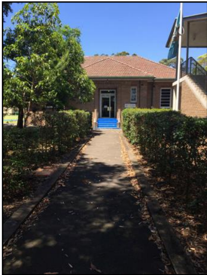
Figure 19. View from the northern boundary to the northern elevation of Building A, facing south. (Source: Heritage 21, 17.01.17)
