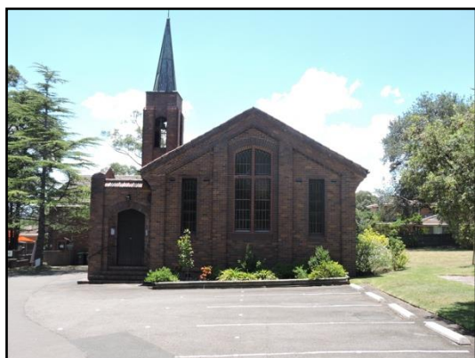
Figure 9. Close-up of the Uniting Church, heritage item 742, from Edgeworth David Avenue, facing north. (Source: Heritage 21, 17.01.17)
