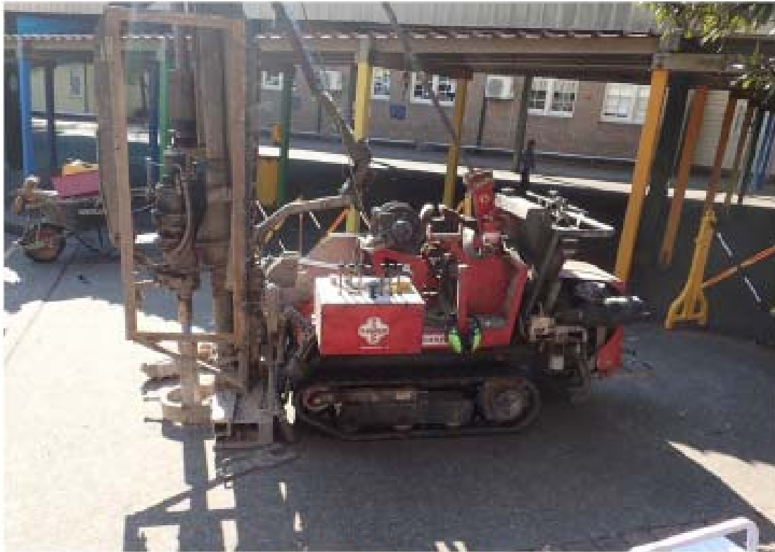
Photo 1 - 1.2 Tonne Tracked Drill Rig
