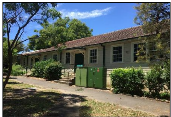
Figure 21. View to the northern elevation of Building J, facing north-east. (Source: Heritage 21, 17.01.17)
