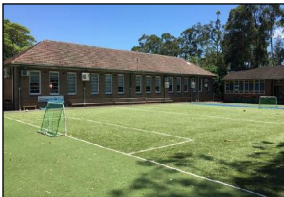
Figure 20. View to the eastern elevation of Building A, facing north-west. (Source: Heritage 21, 17.01.17)
