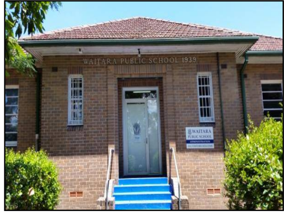
Figure 18. View to the northern elevation of Building A, facing south. (Source: Heritage 21, 17.01.17)
