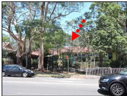
Figure 6. View to the northern boundary of the site, across Edgeworth David Avenue, facing south. Building J is indicated by the red arrow. (Source: Heritage 21, 17.01.17)
