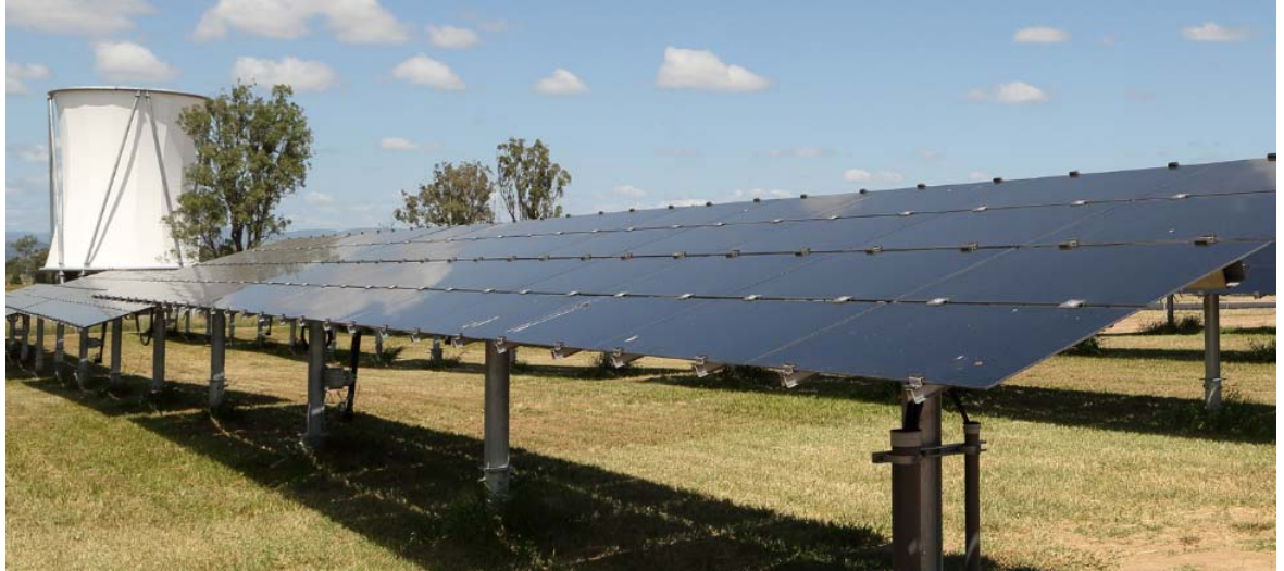
Figure 4-1 First Solar modules and a single axis tracker installed at the Gatton Research Facility in Queensland.
