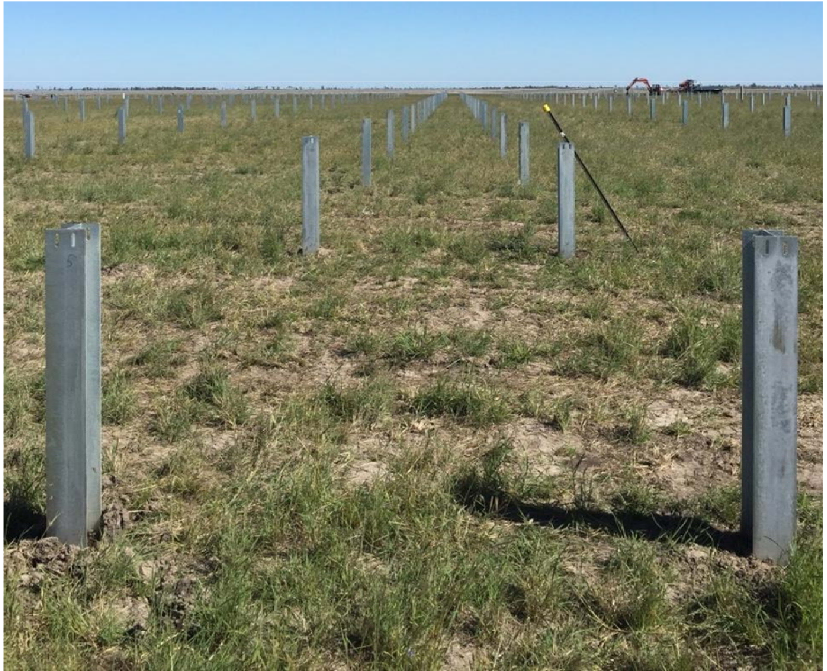
Figure 4-2 Piling installation for a single axis tracker
