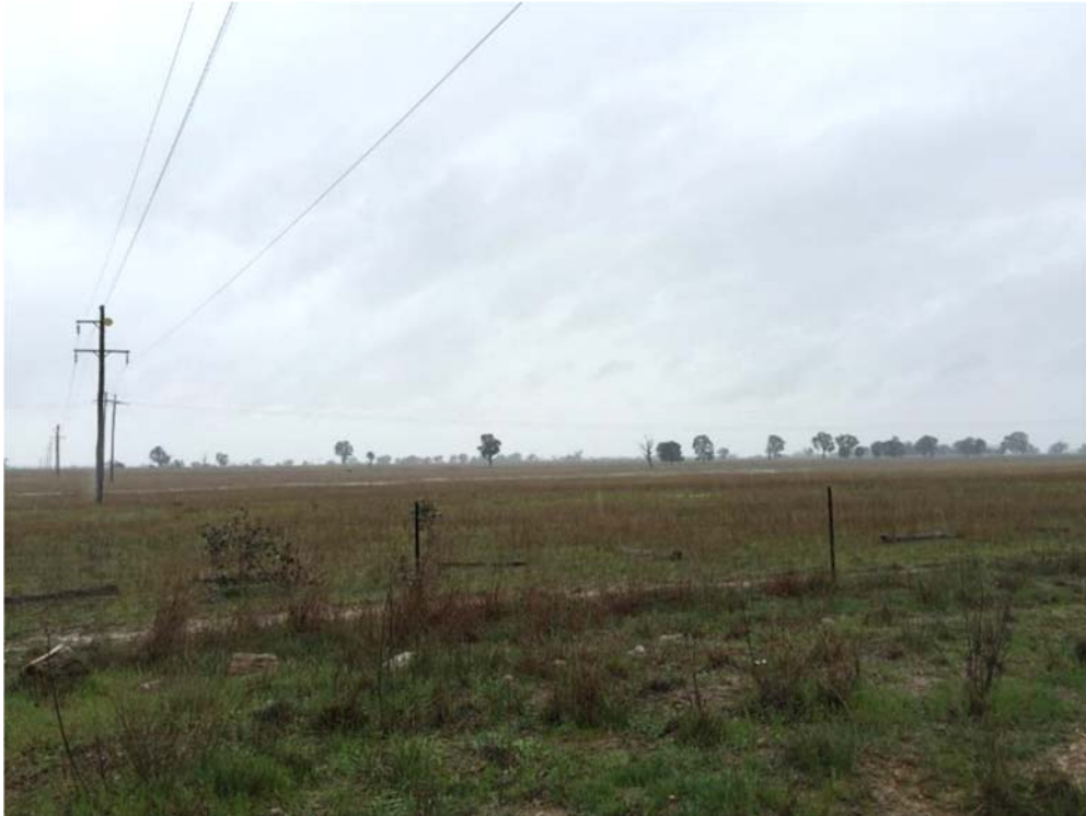
Figure 4-7 Example TransGrid transmission line.
