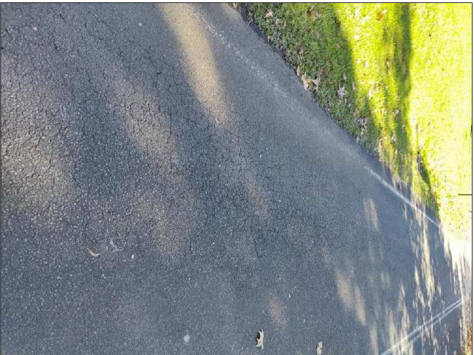
Photo 33: Crocodile cracking
