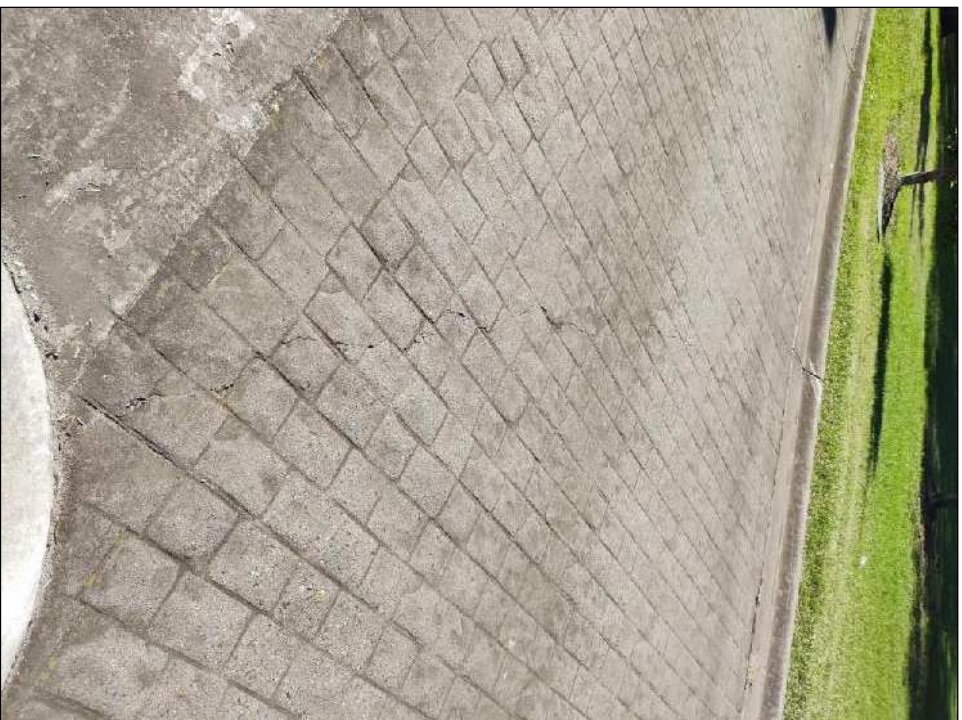
Photo 11: Diagonal crack through pavers
