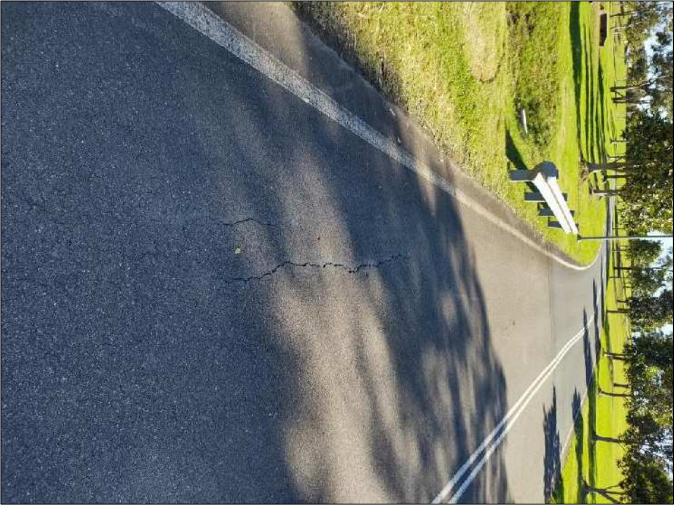
Photo 24: Longitudinal cracking, appears to have been previously ressealed and since opened
