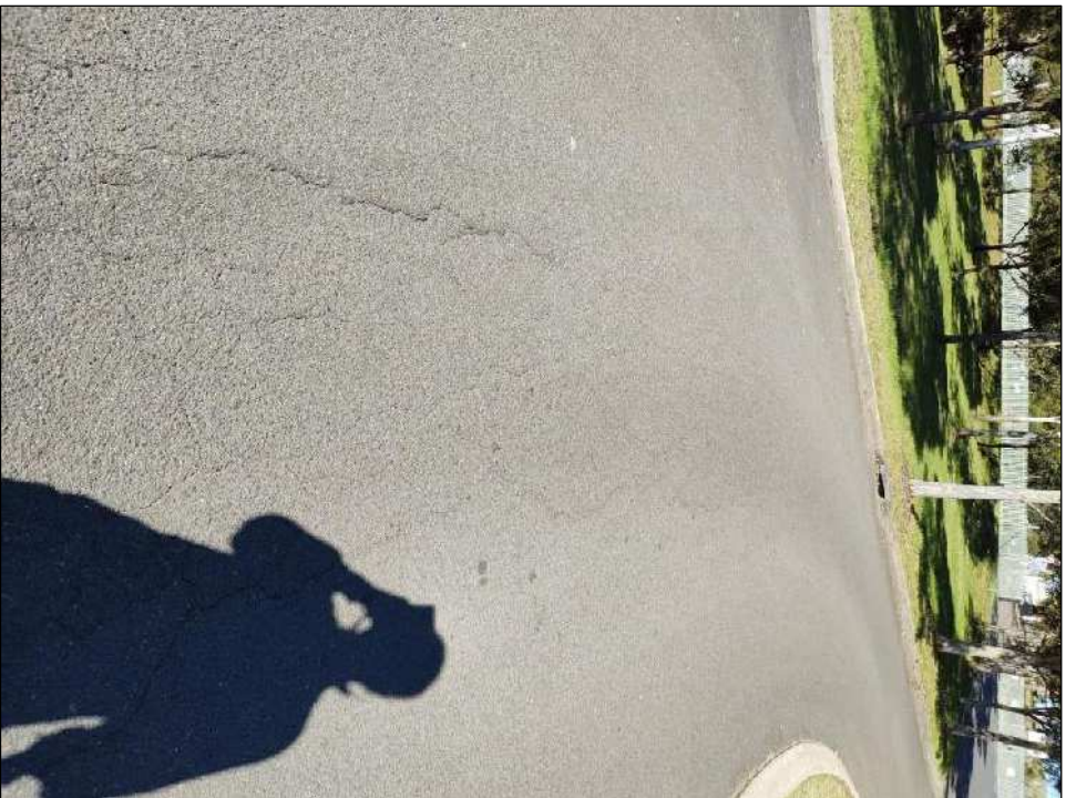
Photo 17: Crocodile cracking, Rutting appearing to occur
