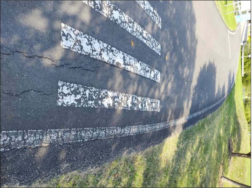
Photo 61: Longitudinal at crossing
