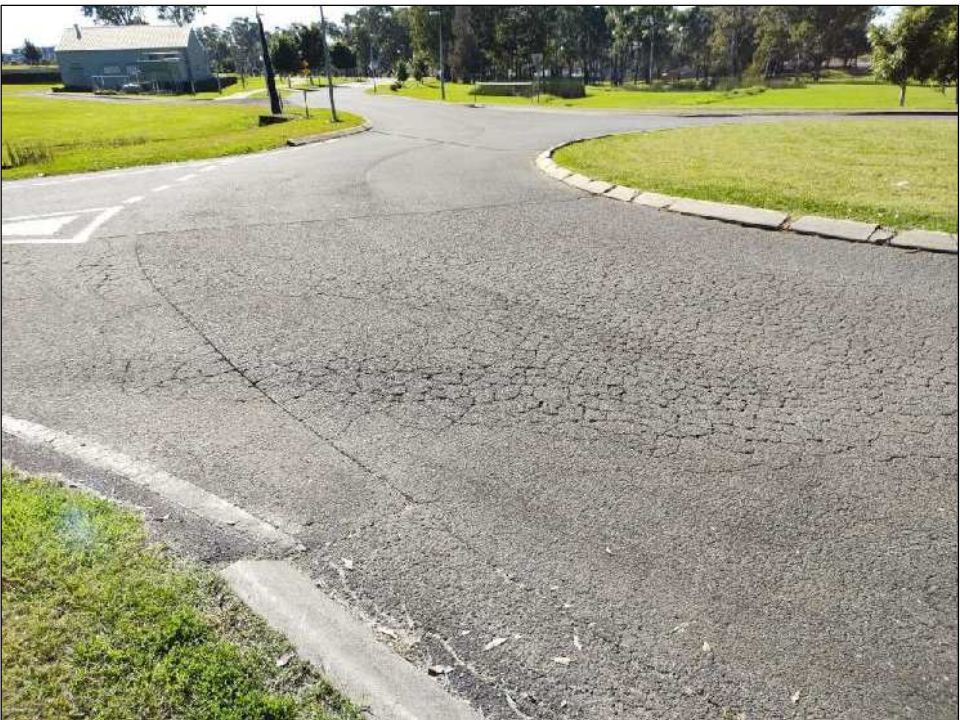
Photo 21: Significant crocodile cracking to the road surface
