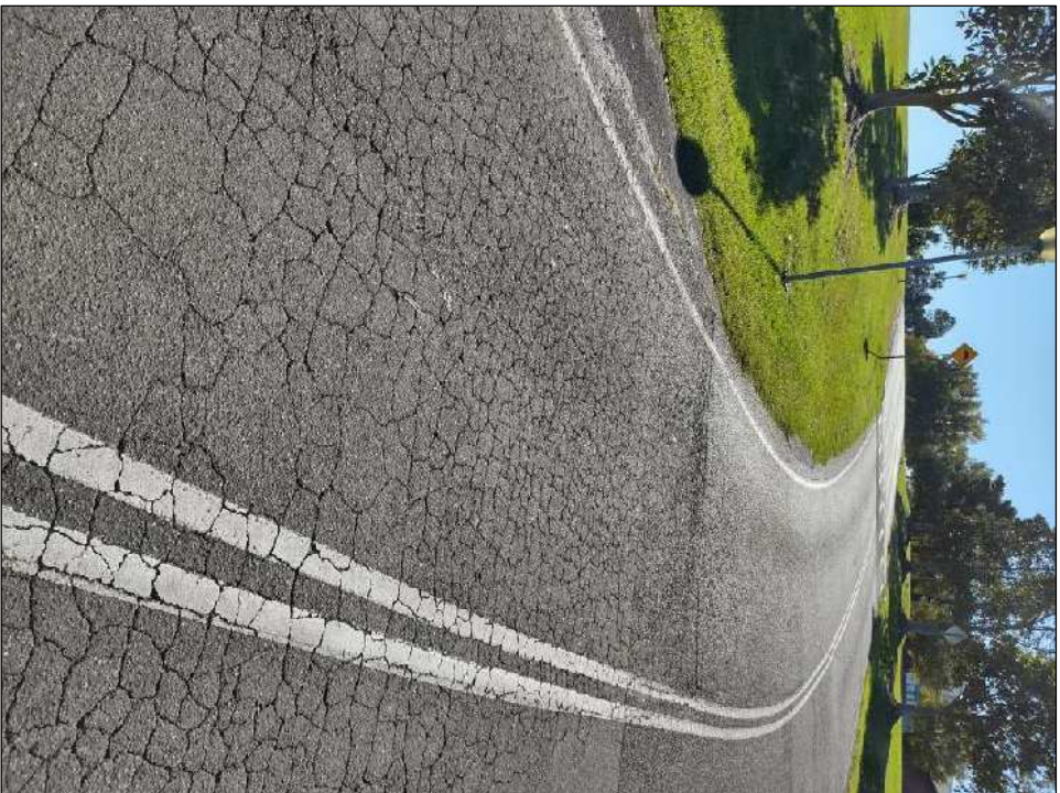
Photo 31: Severe crocodile cracking
