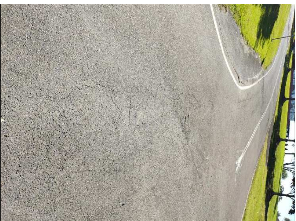
Photo 30: Crocodile cracking and delamination
