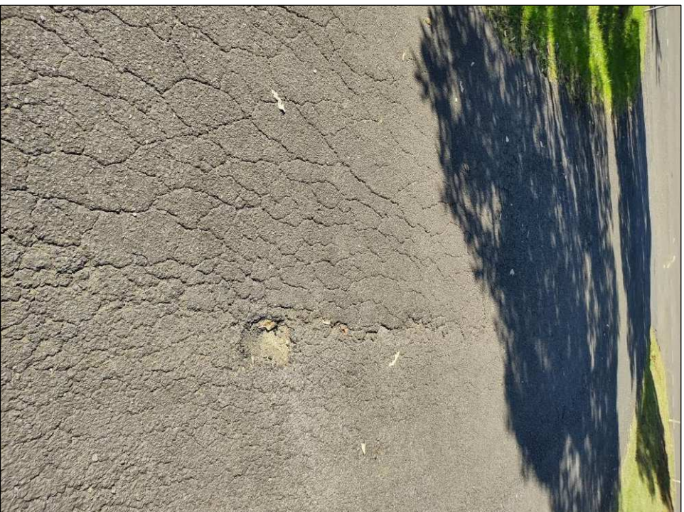
Photo 56: Crocodile cracking, pots holes
