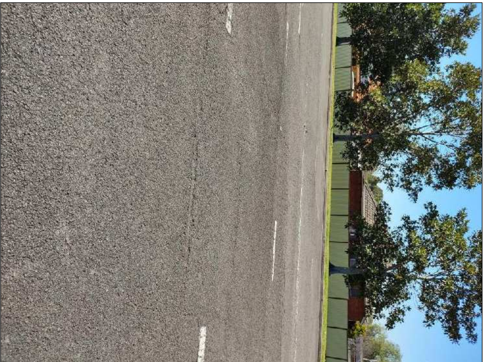
Photo 51: Deformation in the form of crocodile cracking
