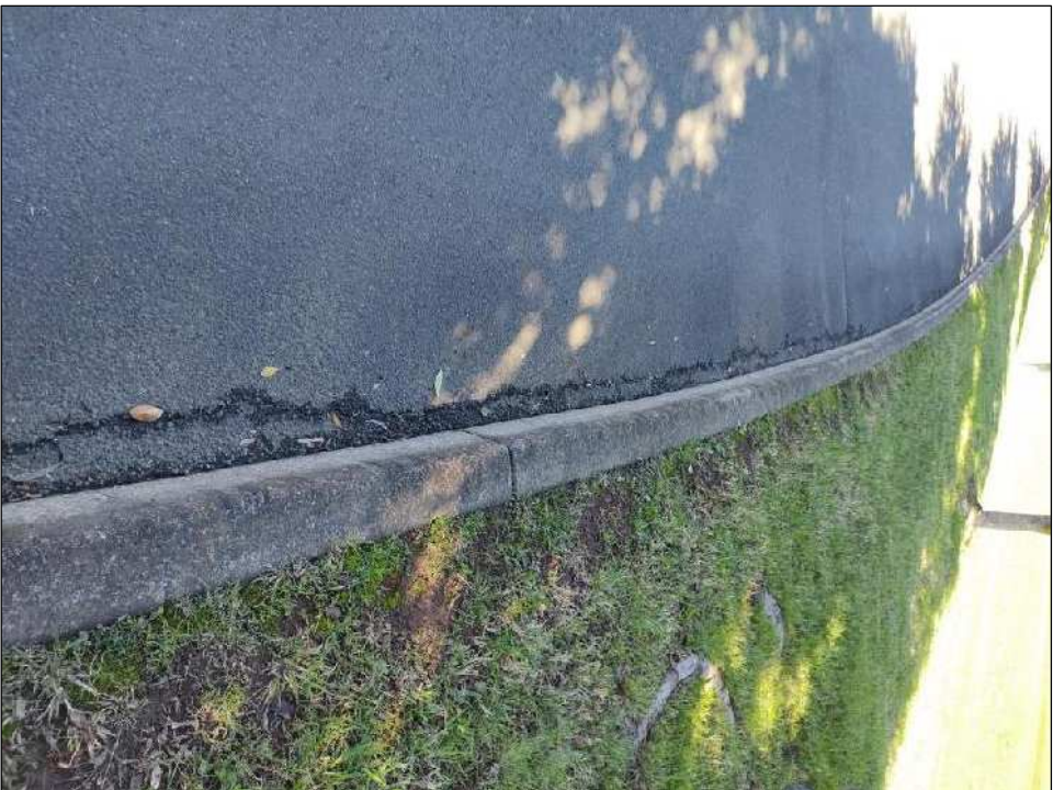
Photo 43: Edge breaks and signs of heaving/shoving??
