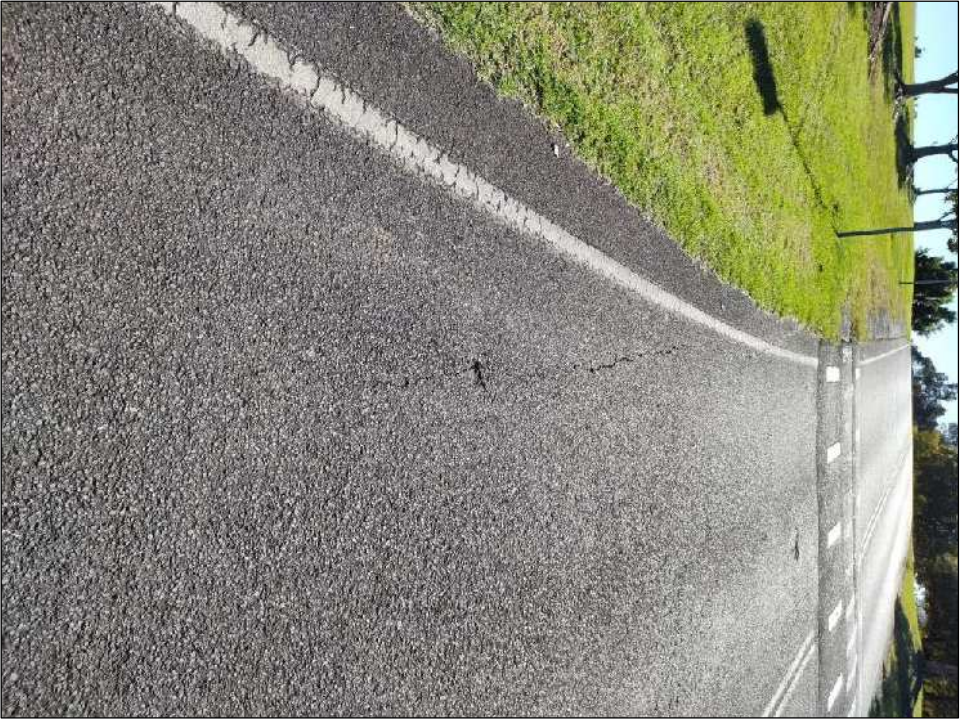
Photo 32: Longitudinal cracking
