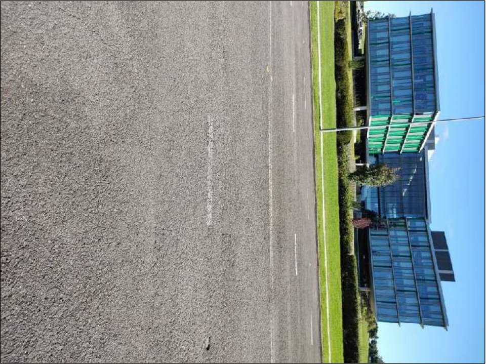
Photo 2: Crocodile cracking, minor patching
