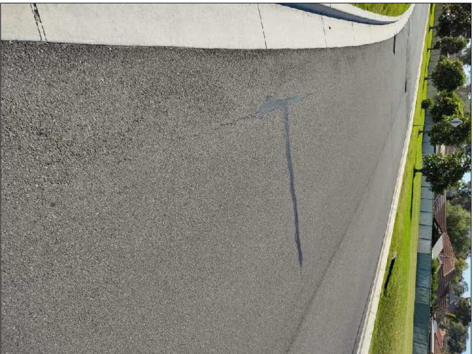
Photo 50: Longitudinal and horizontal crack
