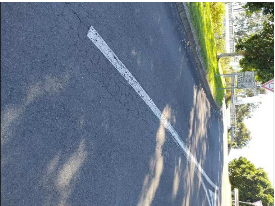
Photo 45: Crocodile Cracking
