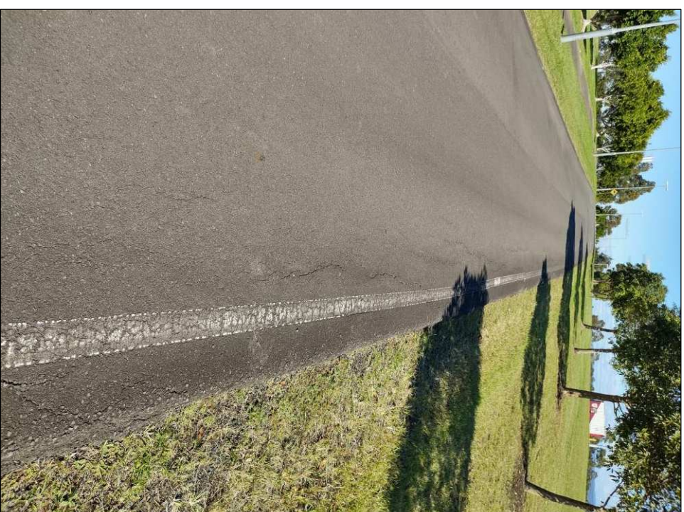
Photo 65: Longitudinal cracking along outer wheel path
