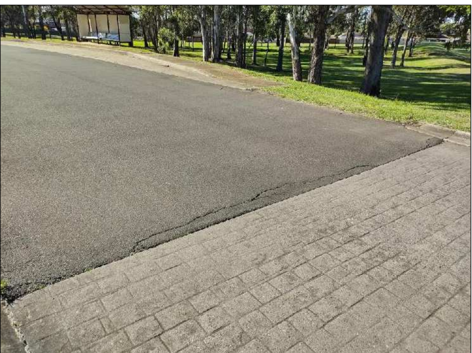
Photo 10: Edge break at construction joint between pavement types
