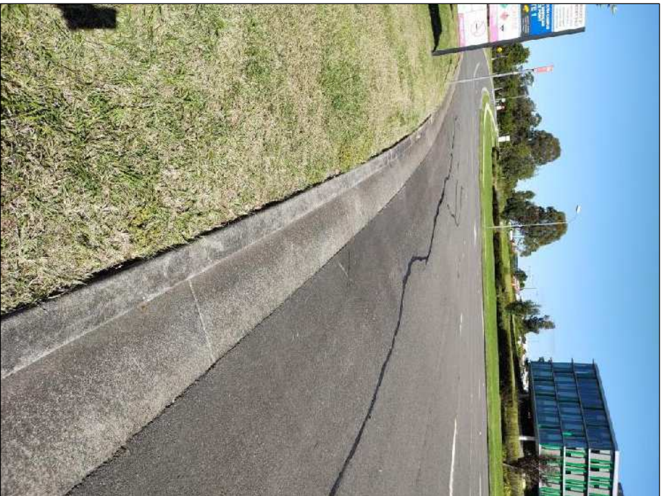
Photo 1: Longitudinal/meandering cracks, previously ressealed
