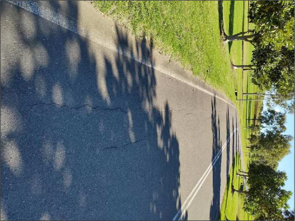
Photo 22: Longitudinal cracking
