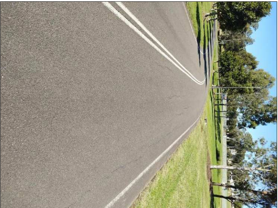
Photo 23: Longitudinal cracking, appears to have been previously ressealed and since opened
