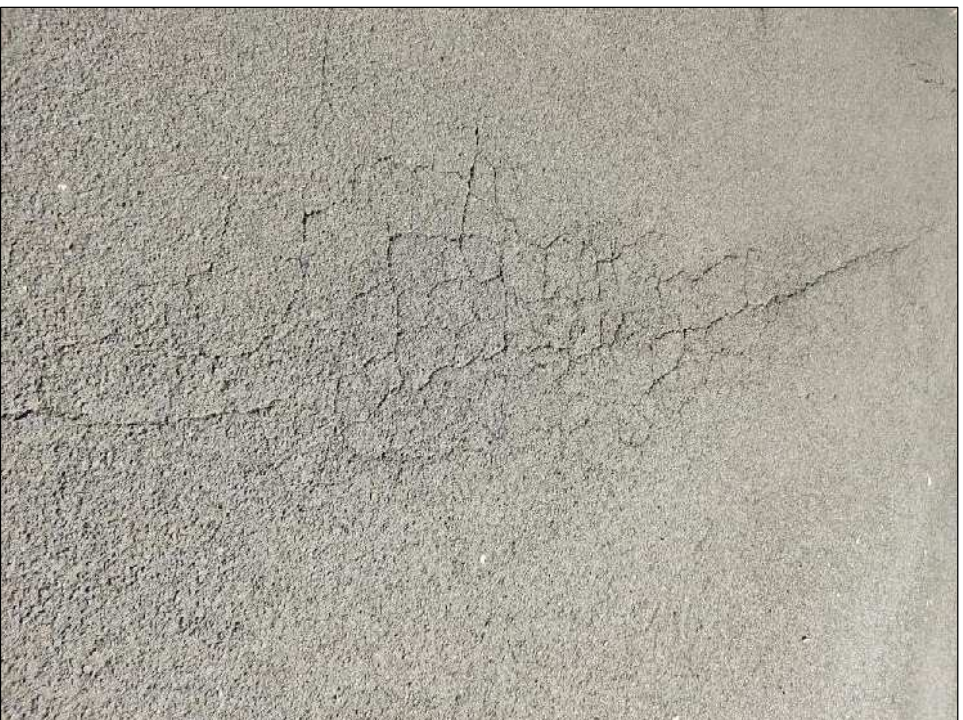
Photo 19: Crocodile cracking
