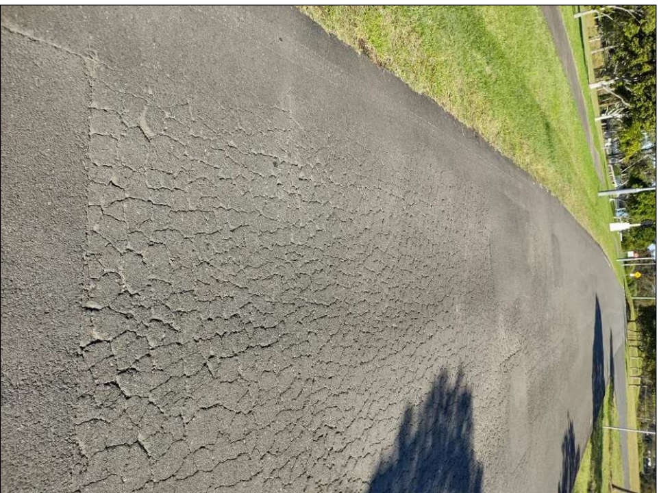
Photo 64: Crocodile cracking and patching
