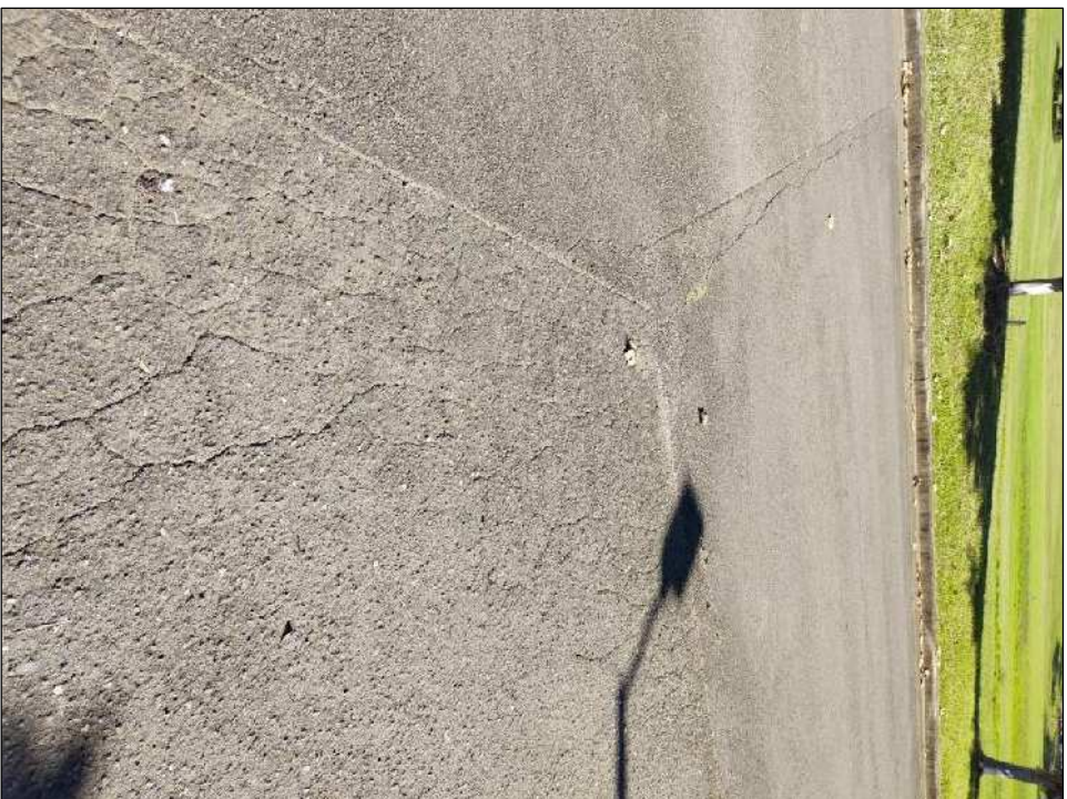
Photo 37: Horizontal crack at junction of resealed section. Crocodile cracking noted on the southbound side of the road
