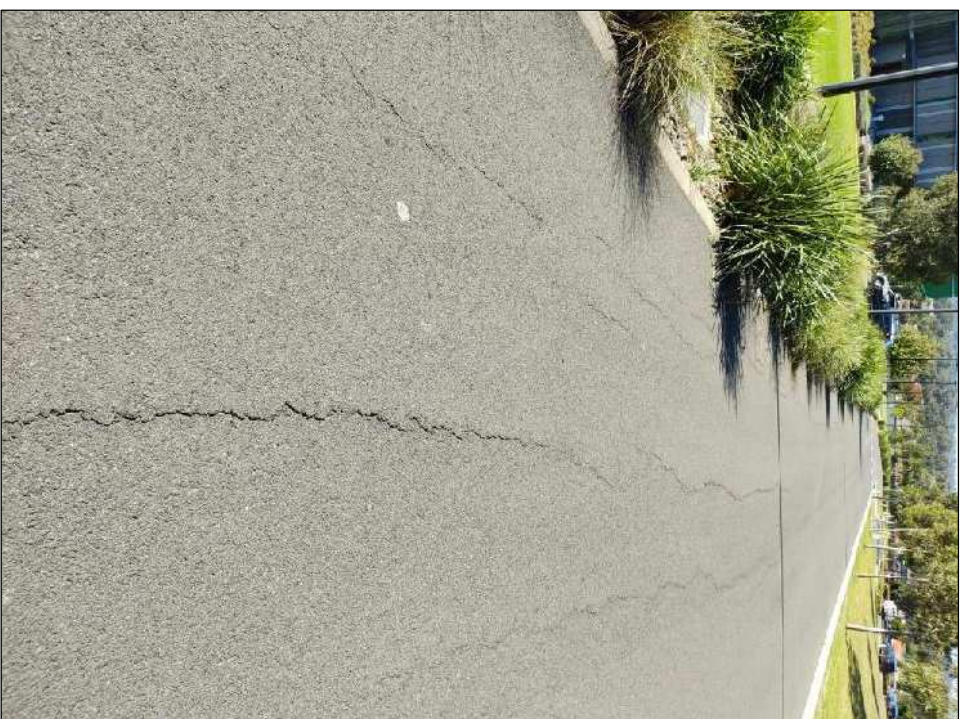
Photo 48: Longitudinal cracking
