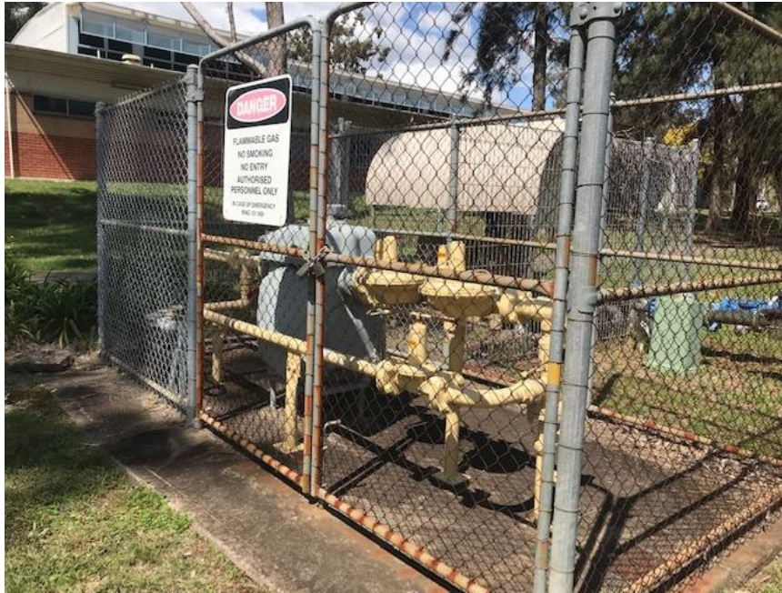
Photo: Existing gas meter (high pressure meter and reg set)
