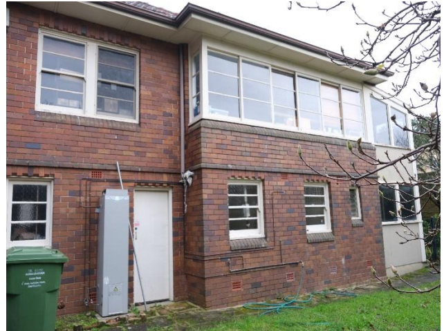
Figure 25 View of rear façade of 25 Rosedale Road, Gordon.
