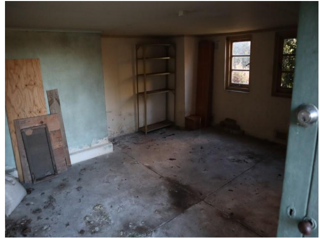
Figure 62 Basement level storeroom.
