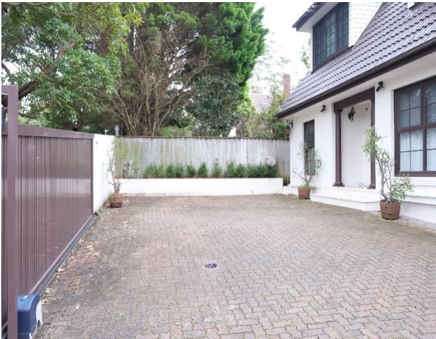
Figure 30 View of front car parking space, facing west.
