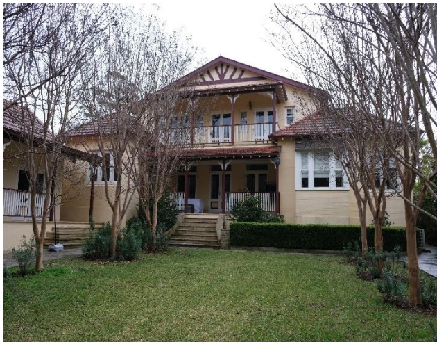
Figure 6 View of the rear façade 1 Edward Street, Gordon.
