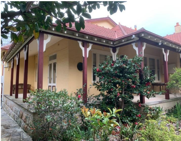
Figure 10 View of the western portion of the primary façade of 1 Edward Street, Gordon.
