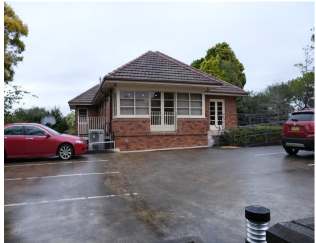
Figure 23 View of southern elevation of 25 Rosedale Road, Gordon.
