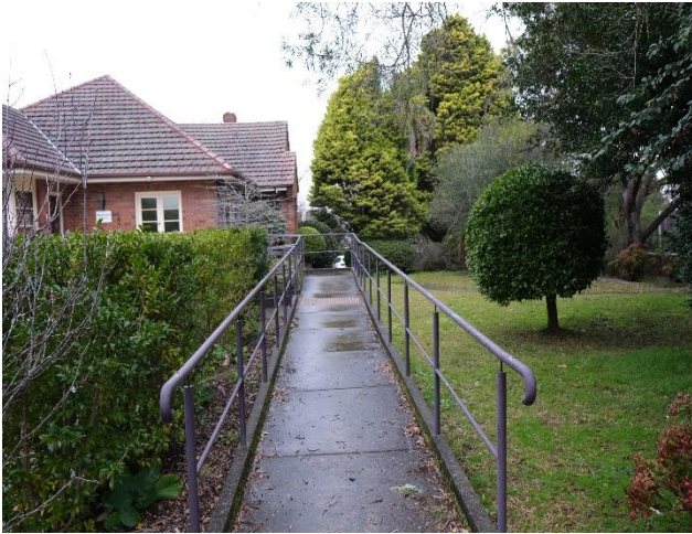
Figure 24 View of primary access point to 25 Rosedale Road, Gordon.
