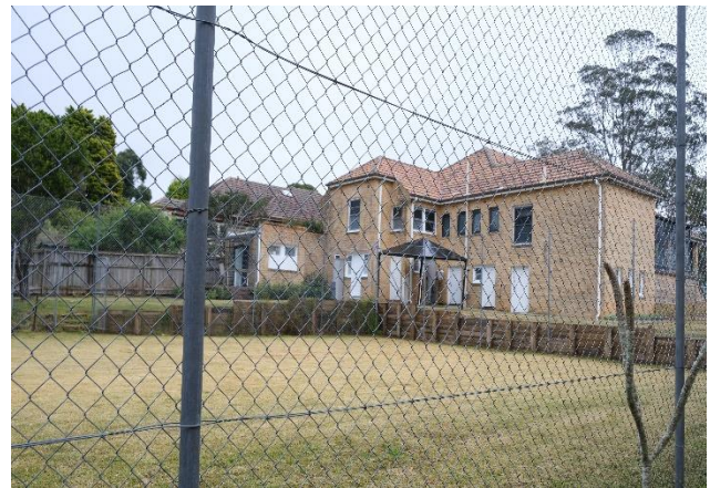
Figure 19 View of rear façade of 1A Edward Street, Gordon.
