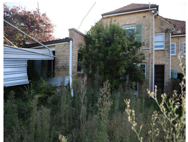
Figure 52 Rear façade and garage.
