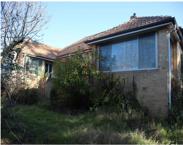
Figure 49 Northern elevation and rear addition.
