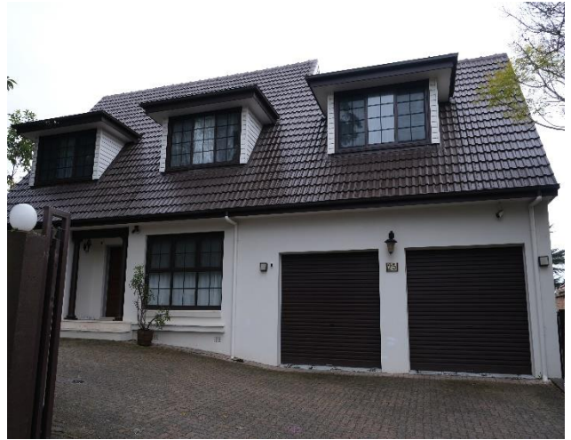
Figure 29 View of primary façade of 27 Rosedale Road, Gordon, facing north.
