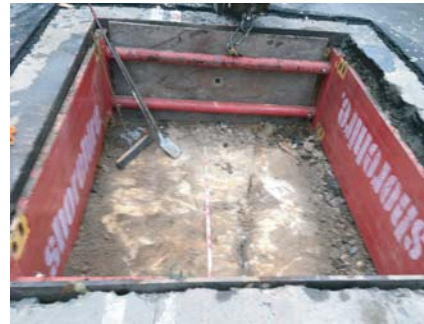
Natural sandstone that has been bench-cut to form a road surface
