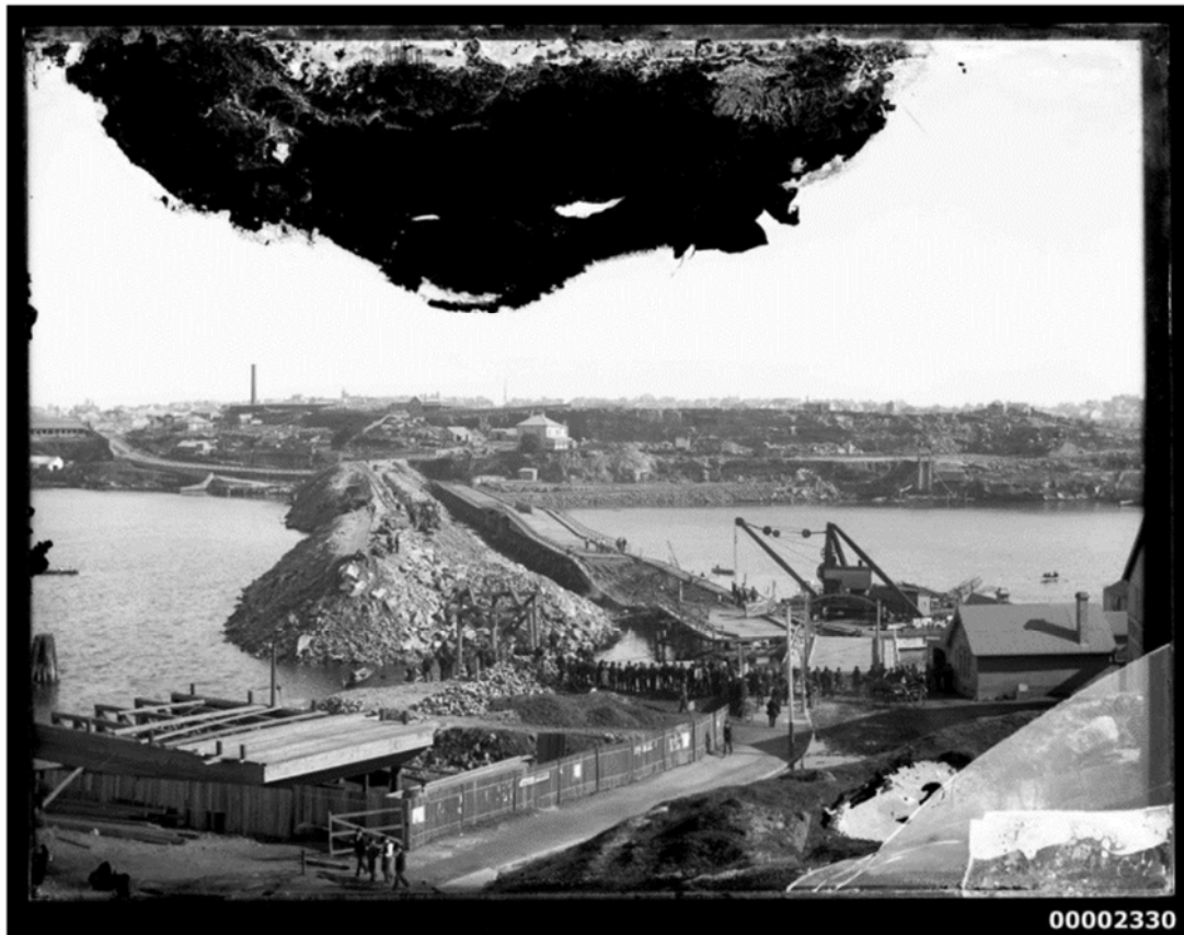
Figure 10 “Glebe Island Bridge collapse” August 1899 (Source ANMM Collection Gift from Bruce Stannard available online)
