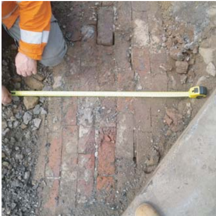
Top of brick barrel drain
