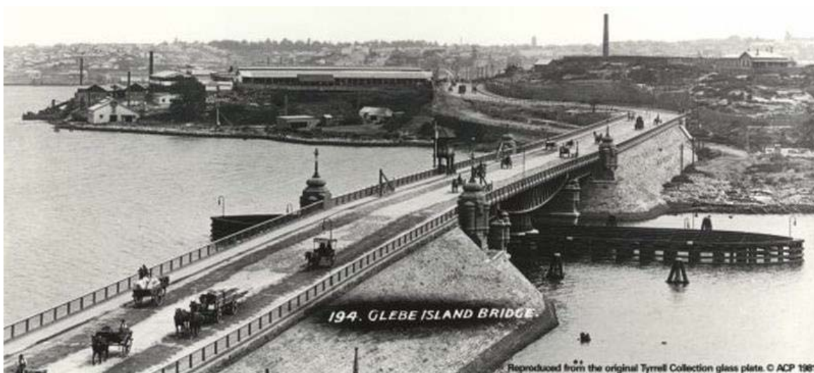
Figure 7 “Glebe Island Bridge c.1910). Note: The pile remains of the first Glebe Island Bridge can be seen cut off near the water level on both sides of the timber fenders associated with the current Glebe Island Bridge. (Source Tyrrell Collection held online at the National Library)
