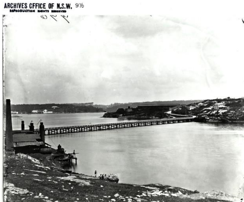
Figure 4 "First Glebe Island Bridge. Glebe (NSW) earlier than 1899 (Source: http://trove.nla.gov.au/version/48145927 )
