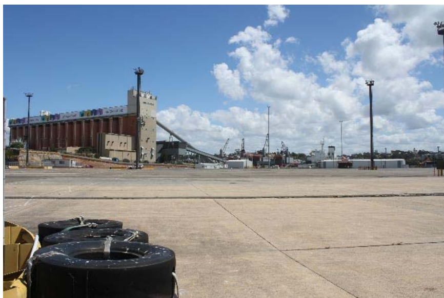
Figure 10 View of Glebe Island Site (View to West)
