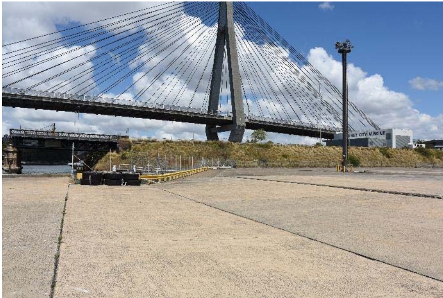
Figure 9 View of the Site on Glebe Island looking towards the western approach of the Glebe Island Bridge. (View to the southwest)
