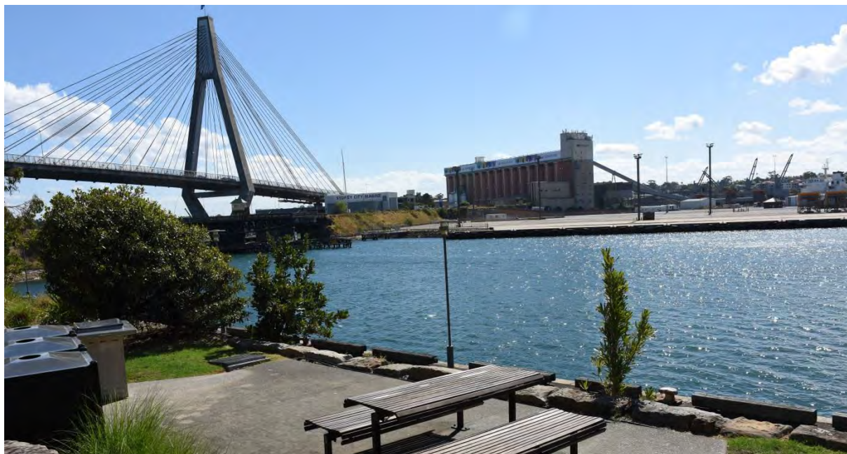
Figure 76 Existing view to the Project site, showing the immediate surrounding development, including the Glebe Island Bridge, Sydney City Marine, The ANZAC Bridge and the existing silos on Glebe Island (Source: AECOM)
