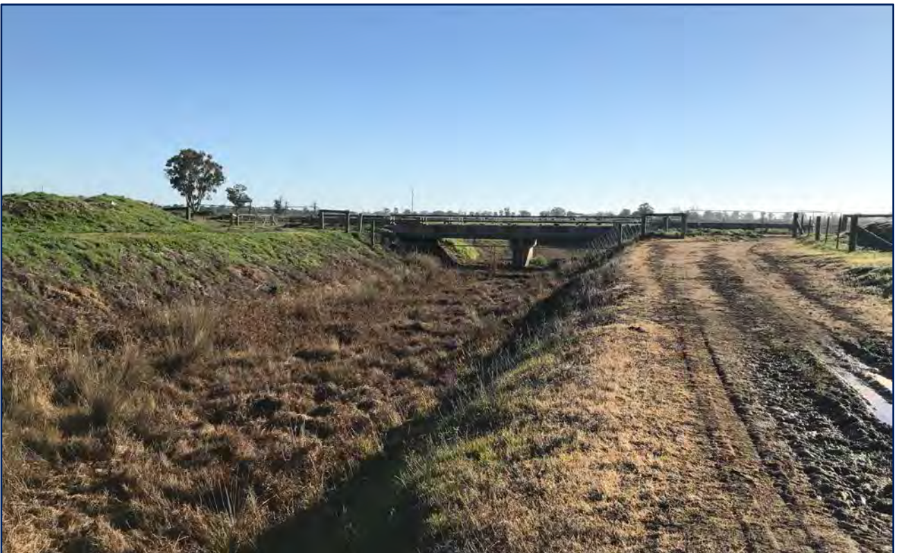
Plate 4 Irrigation channel ULUPNA south of the Broockmanns Road bridge
