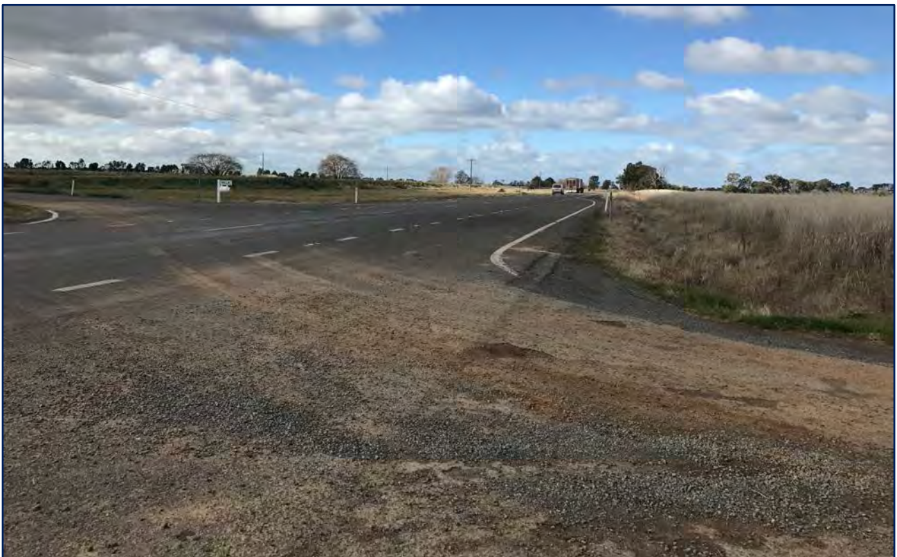
Plate 14 Canalla Road / Riverina Highway Intersection (east)
