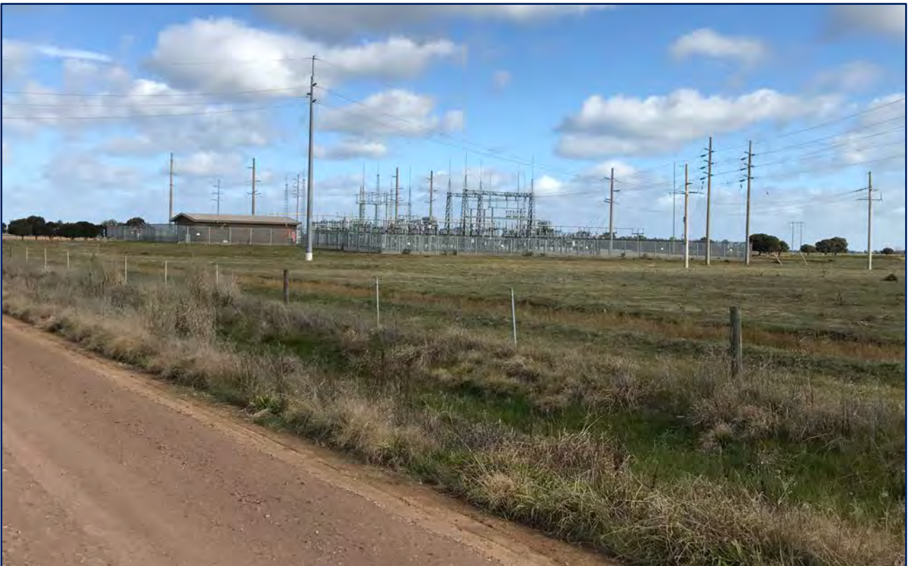
Plate 8 TransGrid's Finley 132 substation and adjoining grazing lands
