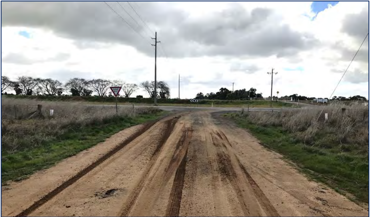
Plate 13 Canalla Road approach to Riverina Highway
