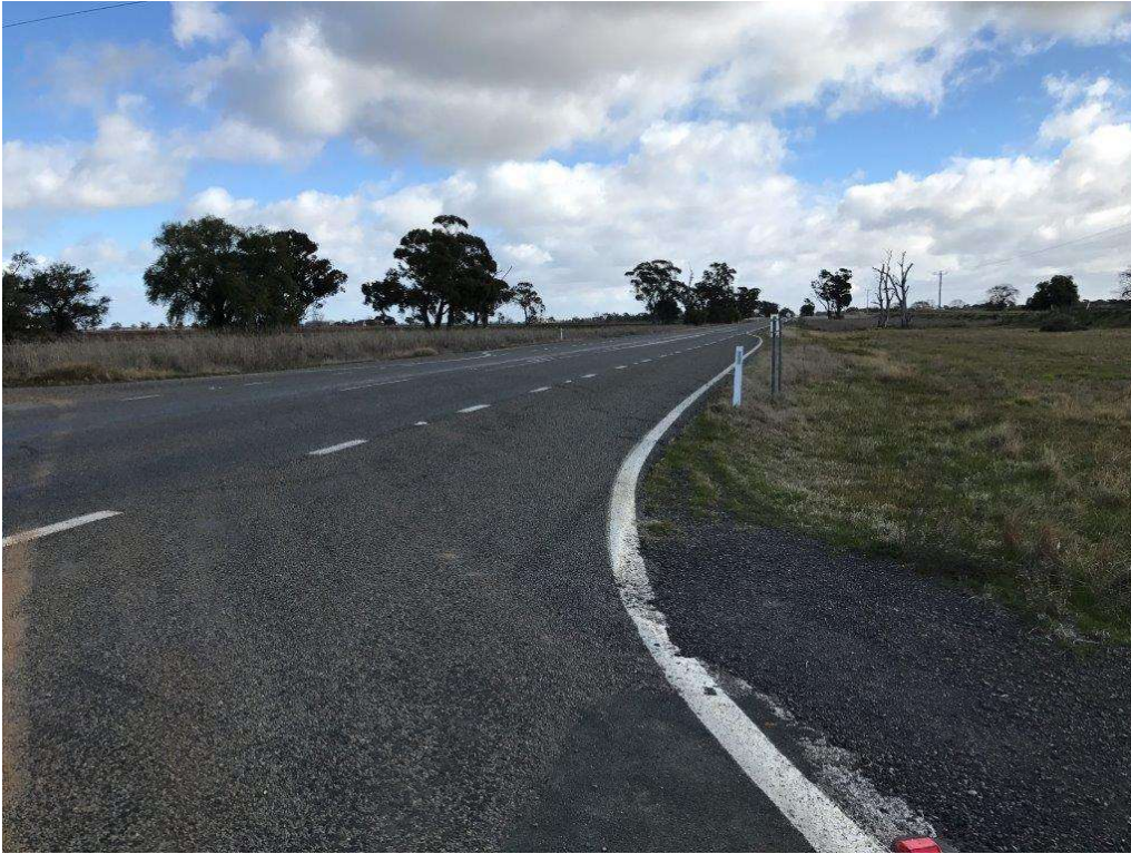
Photograph 4 Marantellis Road / Riverina Highway Intersection looking West
