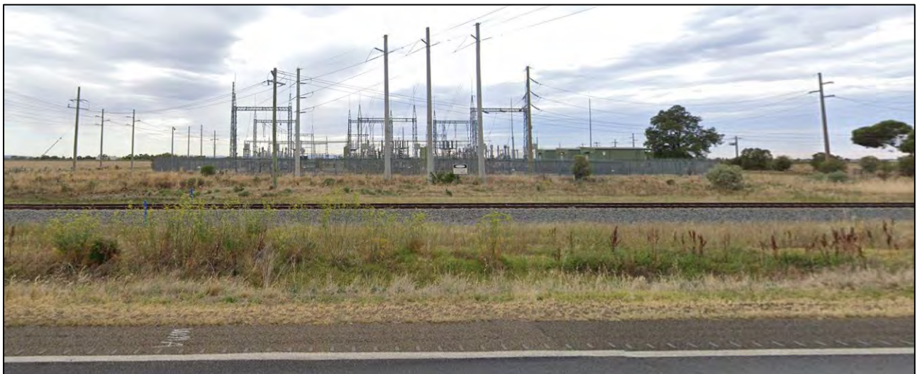
Photo 6: Site conditions of Griffith BESS from Irrigation Way facing north over Griffith Substation with exotic trees. Photo: D.Wall 2024.
