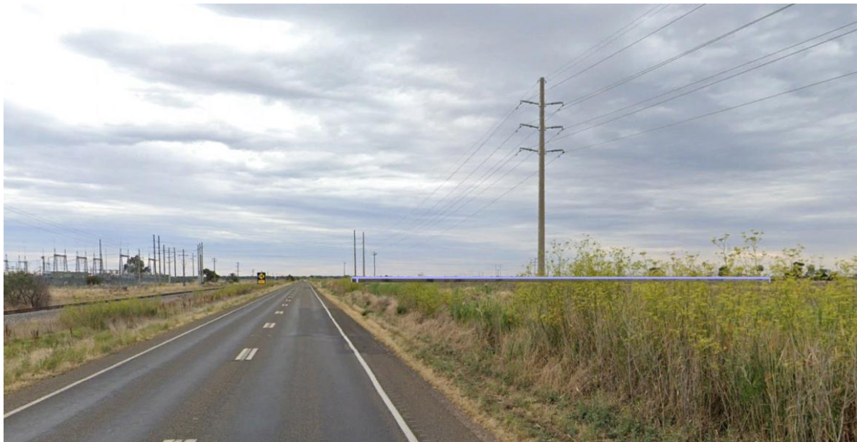
Figure 104 – VP14 – Wireframe view towards the Project only from Irrigation Way. The connecting powerline would be the most visible component (Source: Google Earth Pro).
