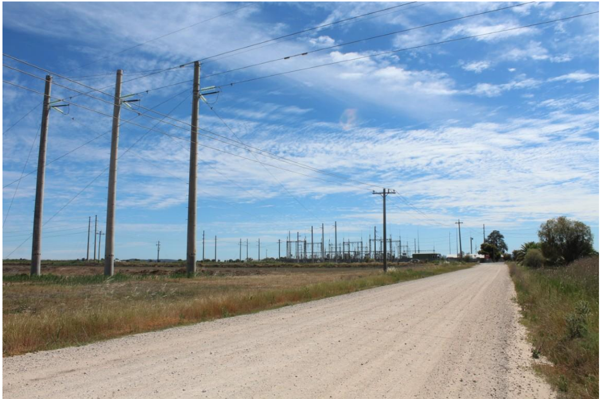
Figure 20 - HV Powerlines traverse the landscape to the north of the Project site as well as adjacent to Irrigation Way from the substation to Yoogali.
