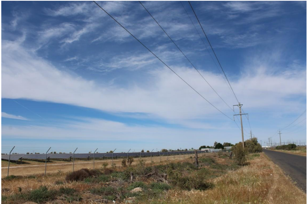
Figure 18 – The Griffith Solar Farm, as viewed from Irrigation Way to the northeast of the Project site.
