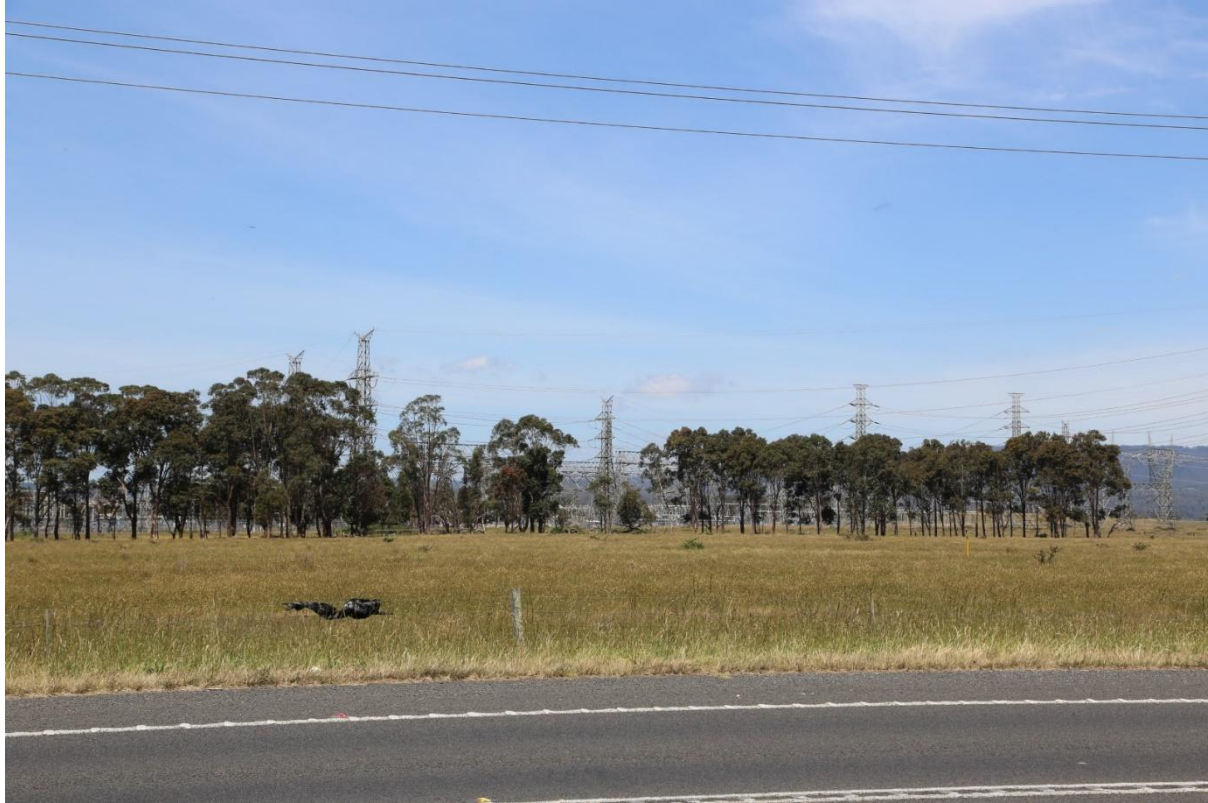
Figure 121 - Example of canopy vegetation providing visual integration of substation infrastructure.
