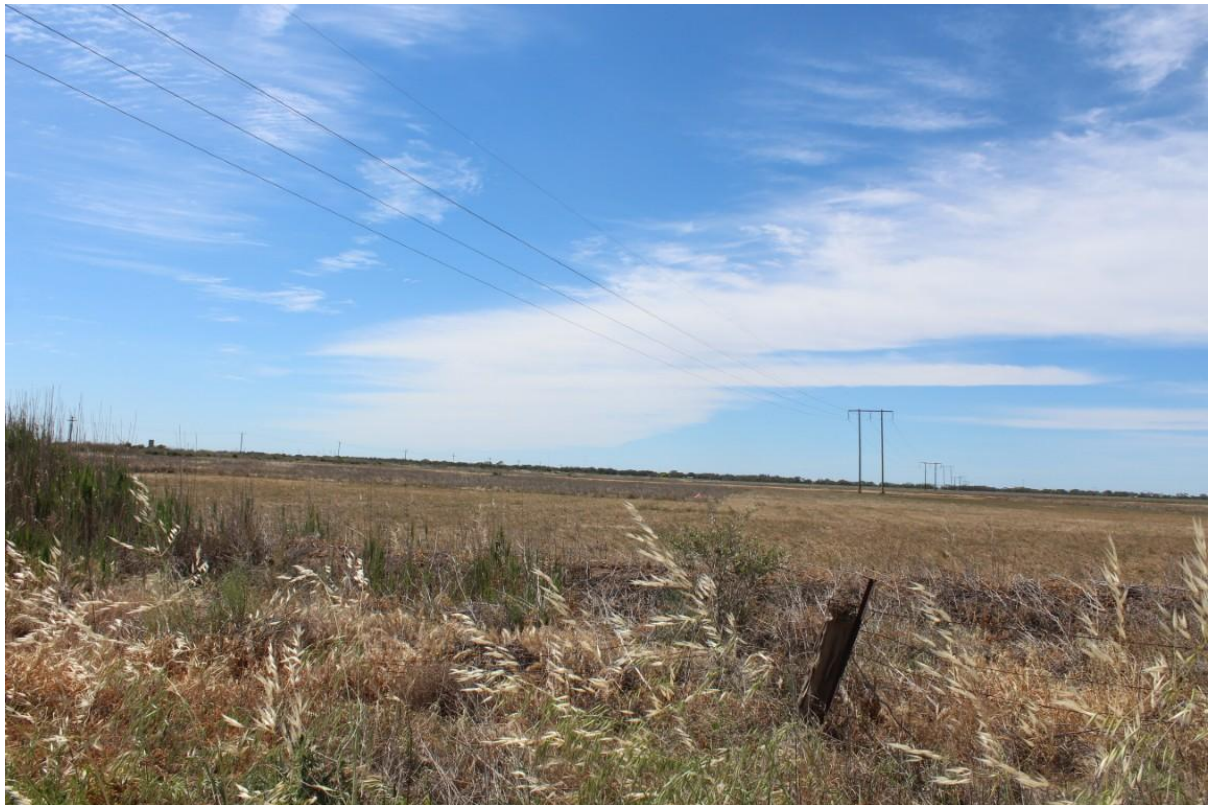
Figure 21 - Existing 33kV power lines run between the Project site and the Yoogali Solar Farm.
