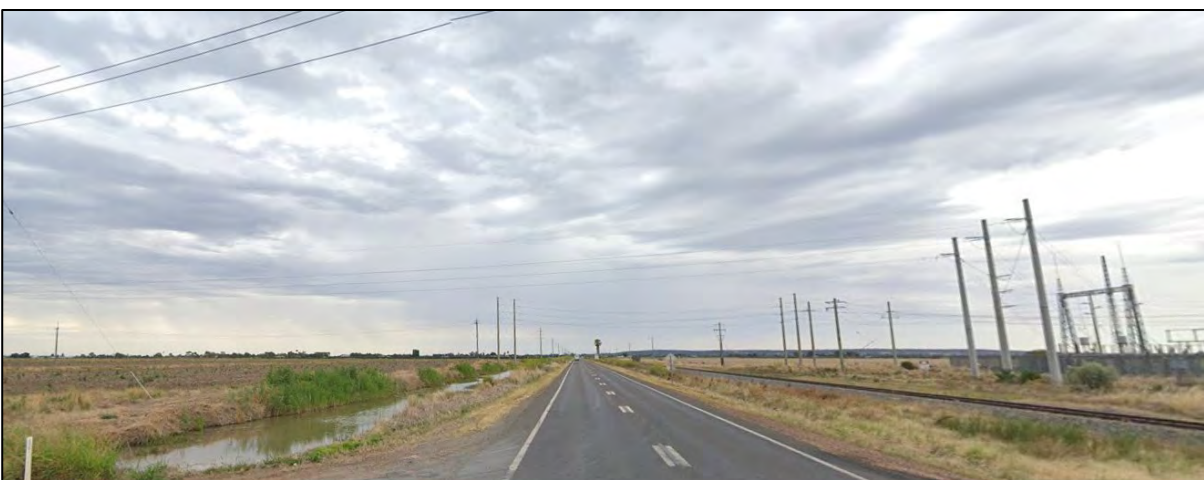
Photo 8: Site conditions of Griffith BESS from Irrigation Way facing north east with Griffith Substation. Photo: D.Wall 2024.
