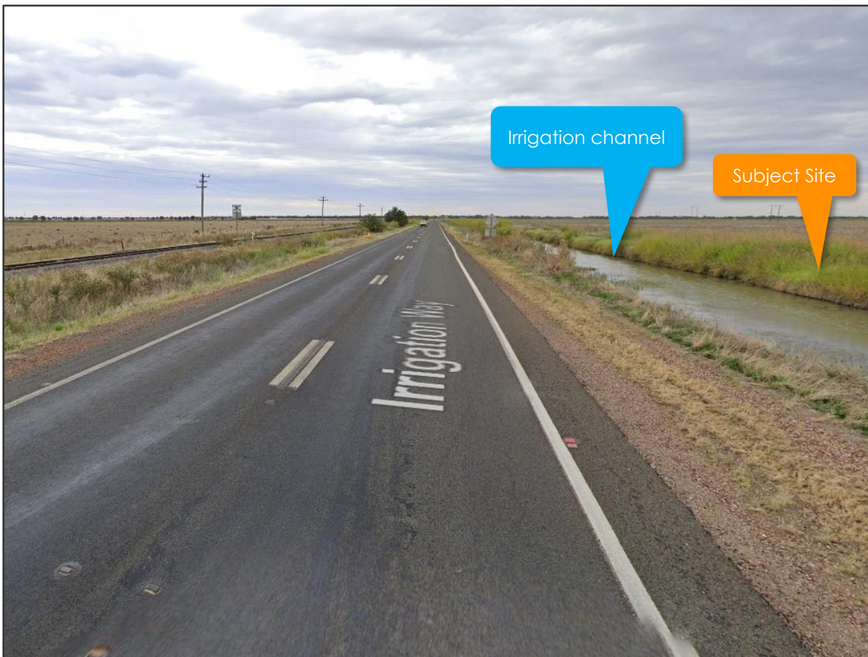
Figure 2 Irrigation Way, looking east adjacent to the site
