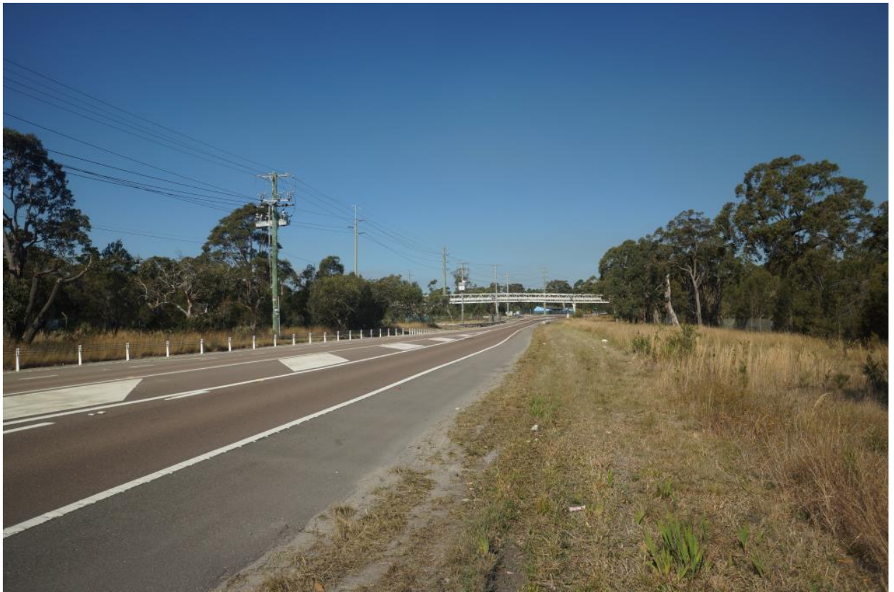
Viewpoint 4 : Network Connection Crossing (looking south east)
