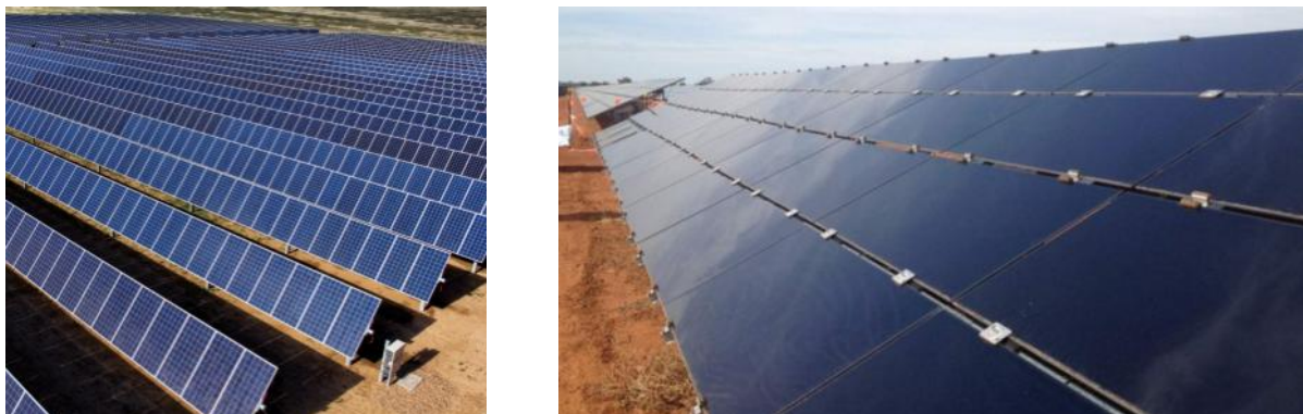
Figure 1.3 : Single axis tracking system (left) and fixed tilt system (right)
