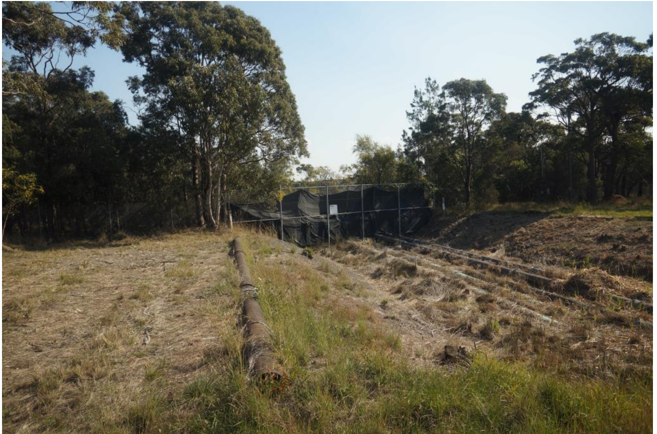
Viewpoint 3 : Ash Delivery Pipes
