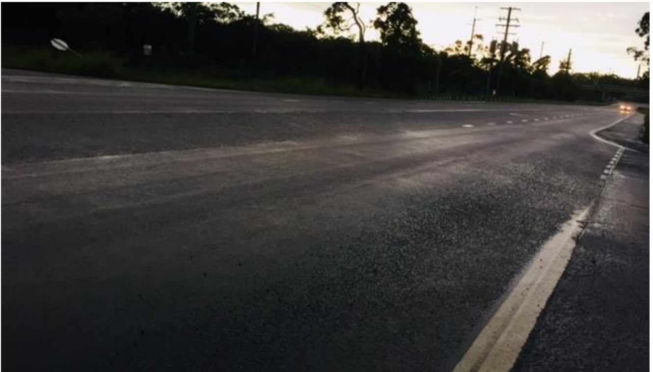
Figure 2-2: Ruttleys Road looking East
