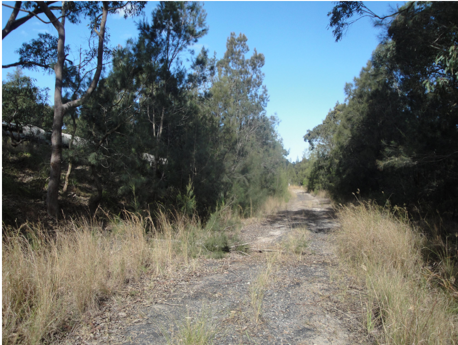
Figure 5.2 : Road construction has brought in imported fill.
