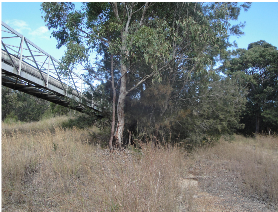
Figure 5.1 : View to south of assessment area exhibiting significant disturbance from conveyor belt and road construction
