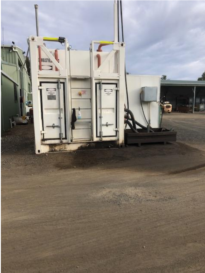
Figure 9. The above ground fuel storage and refuelling area. Visible is an area of localised surface spill
