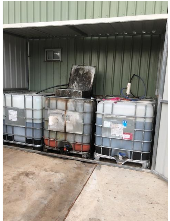
Figure 24. Wastes are pumped out of pit and collected in waste tanks and disposed of off-site by a disposal company
