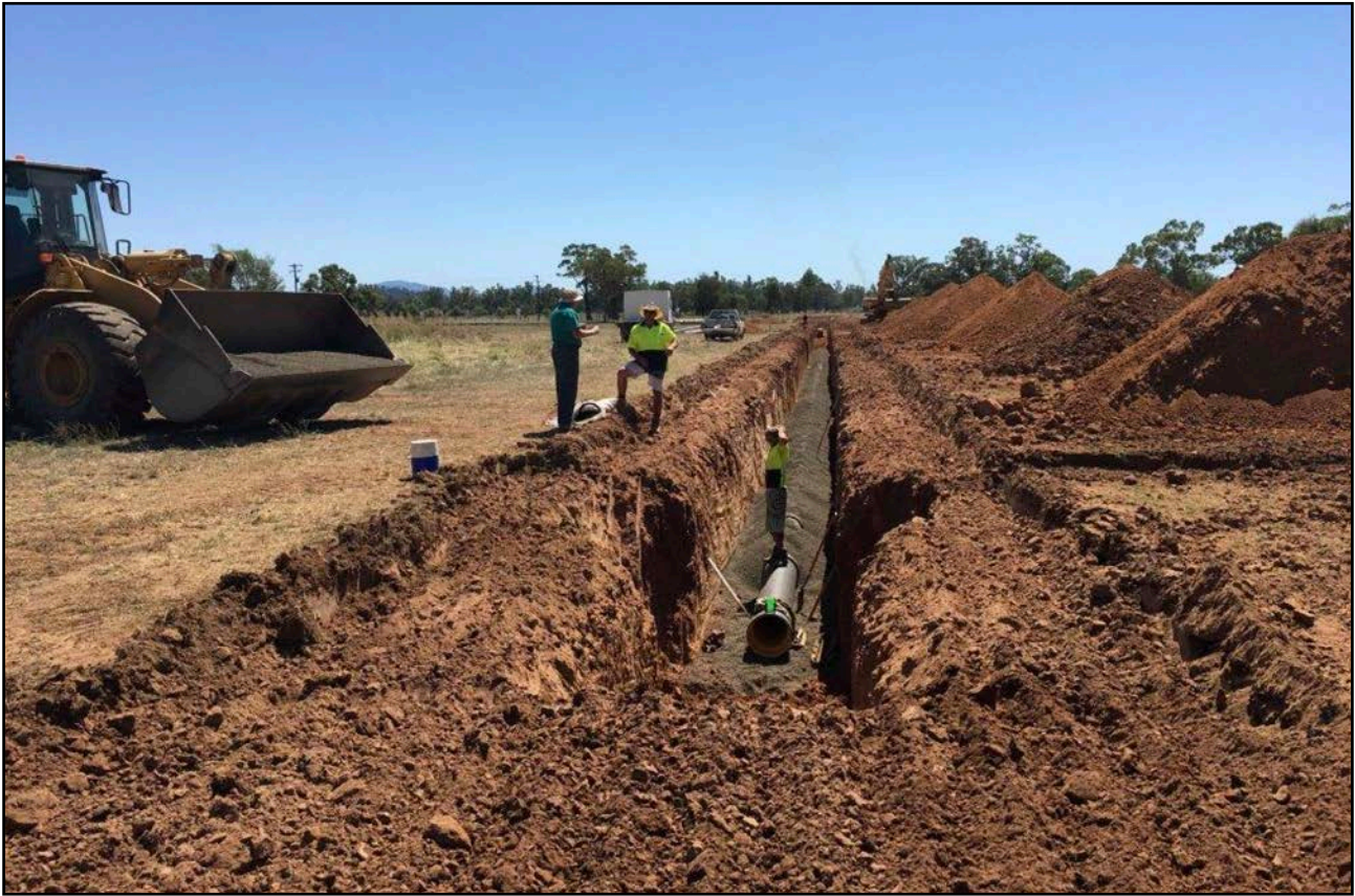
PHOTOGRAPHS 4.1 & 4.2 (above, below): Laying of services for ‘Costalot’ industrial subdivision 2016 on the project site.
