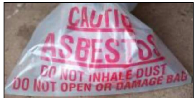
PHOTOGRAPH 3.3 (above): Typical sealed asbestos waste.
