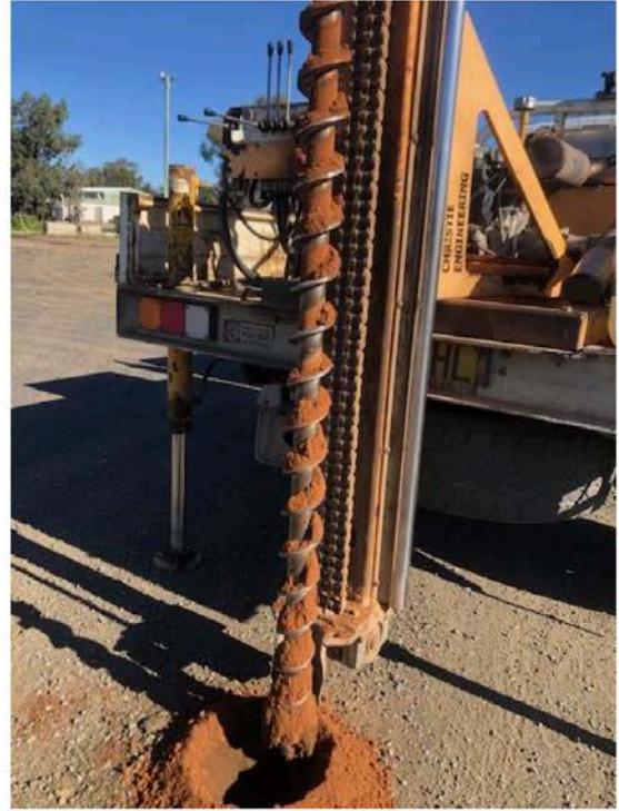
Figure 34. SP10 borehole displaying dry, natural soil beneath 100mm of road base
