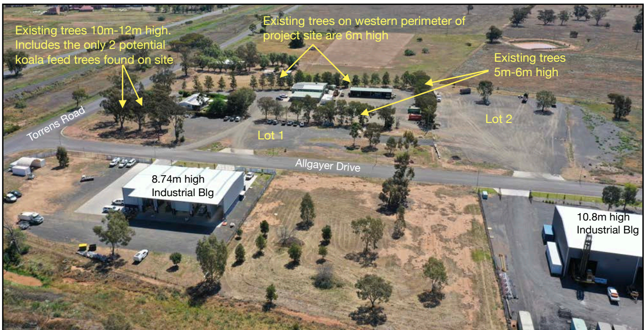
PHOTOGRAPH 4.9 (above): Oblique aerial view of project site with neighbouring industrial and rural land. The project site enjoys well established on-site landscaping.
