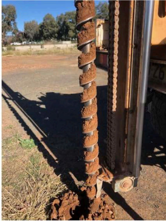
Figure 33. SP9 borehole displaying moist, natural soil beneath 50mm of road base
