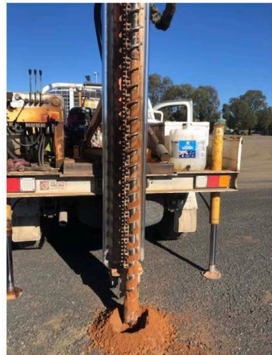
Figure 36. SP12 borehole displaying dry, natural soil beneath 100mm of road base
