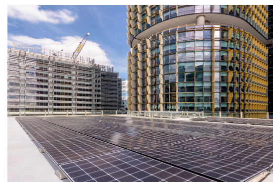
Photo voltaic Panels to Generate Renewable Energy
